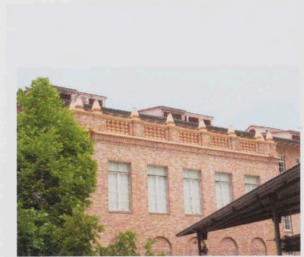
Rooftop terrace on south side of Welch
