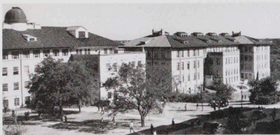
Physics and Chemistry Buildings
