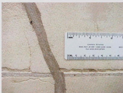
Crack repair
