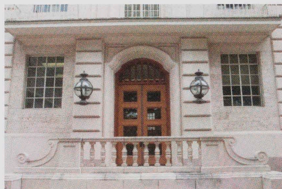
North entrance to Batts, with globe light fixtures
