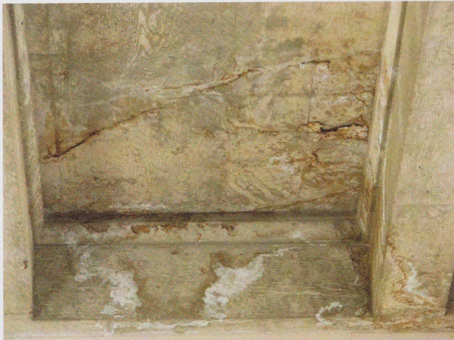
Deteriorated concrete on the ceiling of the Goldsmith loggia
