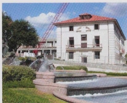
BEN-MEZ hyphen under construction in 2004
