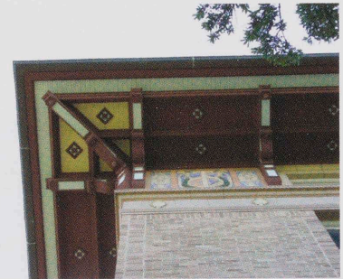
Painted wooden soffits on Sutton Hall
