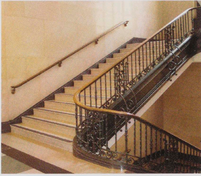
Ornamental iron and bronze stair railings at main stairway
