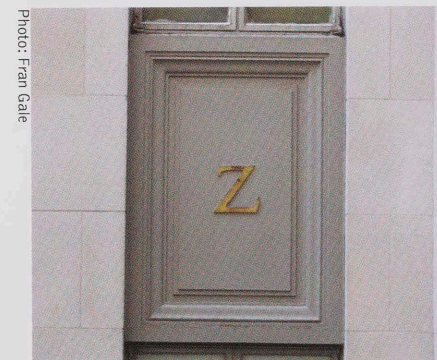
Photo: Fran Gale Main Building Tower painted cast iron spandrel panels, featuring gold lettering
