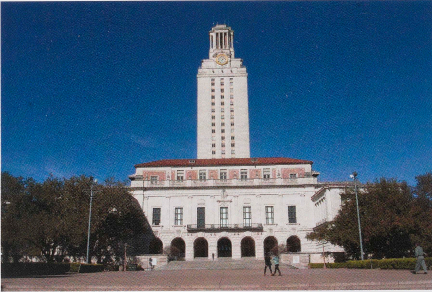
Main Building and Tower, 1937 (contributing, H-1)
