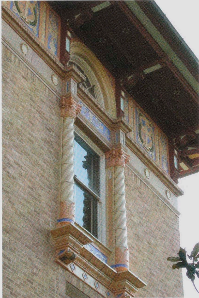
Decorative terra cotta features on exterior and decorative overhanging eave with brackets
