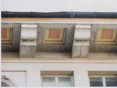
Concrete soffits on the Main Building
