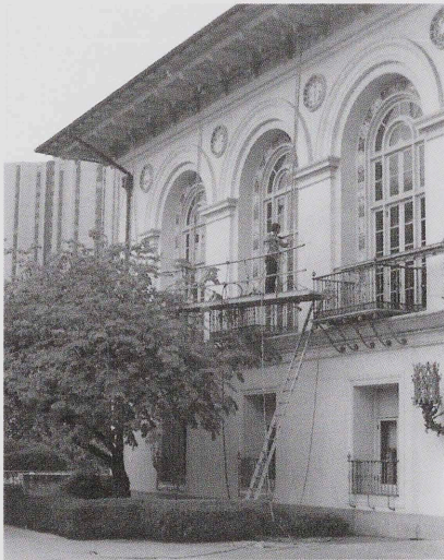
Water blasting of Cordova Cream exterior of Battle
