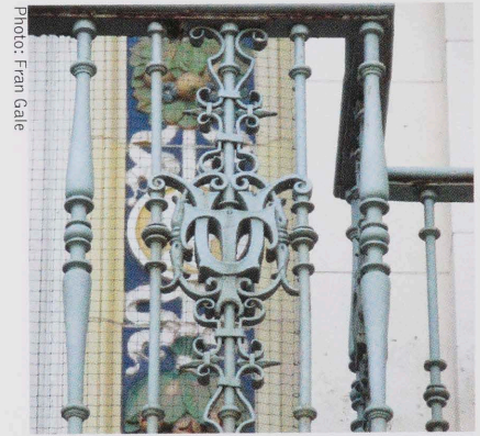
Photo: Fran Gale Intricate wrought iron balcony over Battle Hall entrance, depicting "UT" design
