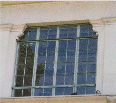
Steel casement windows on Goldsmith Hall. Goldsmith has a combination of wood and metal windows
