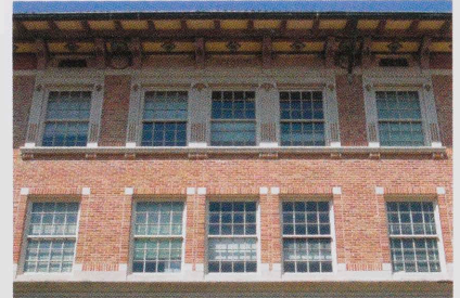
Terra cotta ornamentation and decorative soffit
