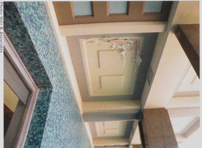
Peeling stucco on the ceiling of the fourth-floor loggia of Flawn
