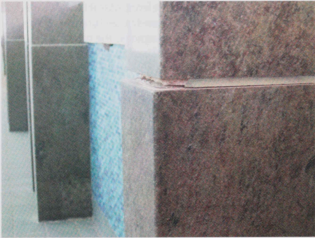
Displacement of meta-anorthosite on the west façade
