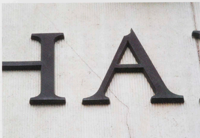
Limestone cracks behind bronze lettering
