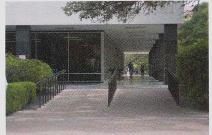
First-floor colonnade and storefront walls
