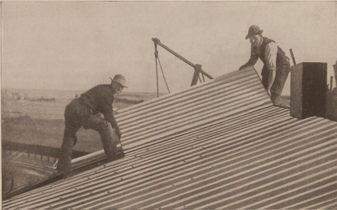
Applying Ambler Asbestos Corrugated Roofing on Steel Structure
