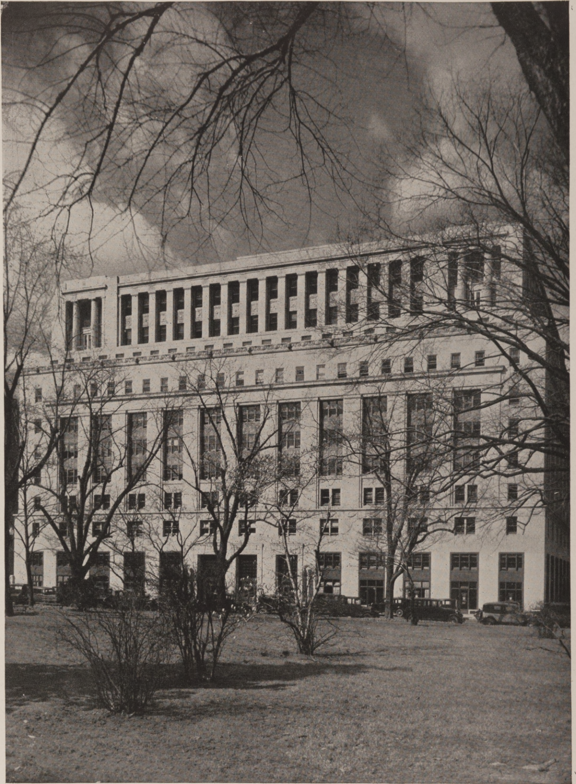
THE SOUTHERN RAILWAY BUILDING, WASHINGTON, D. C. WADDY B. WOOD, ARCHITECT
