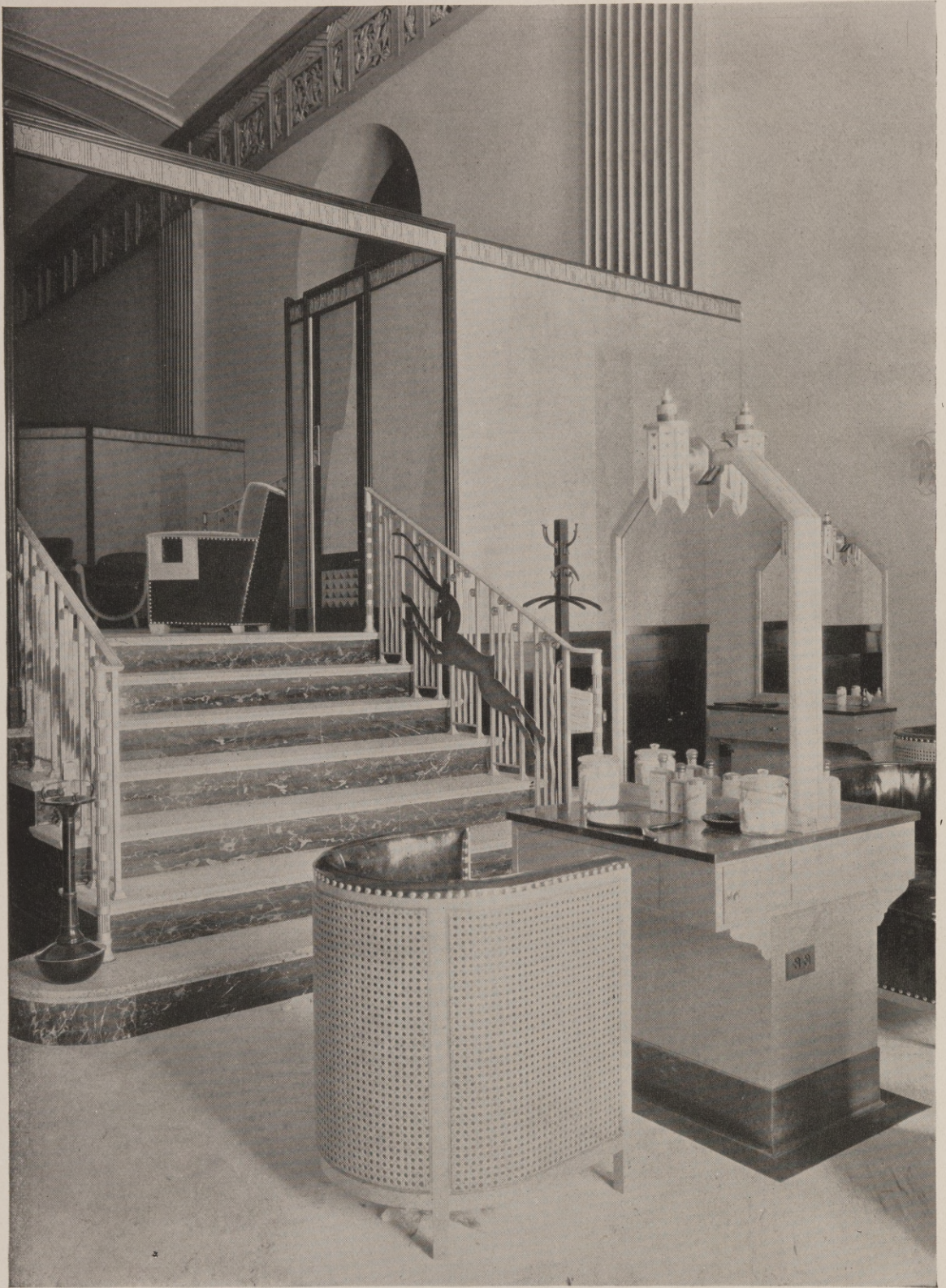
DETAIL IN BEAUTY SALON THE NEIMAN-MARCUS DEPARTMENT STORE, DALLAS, TEXAS GREENE, LAROCHE & DAHL, ARCHITECTS
