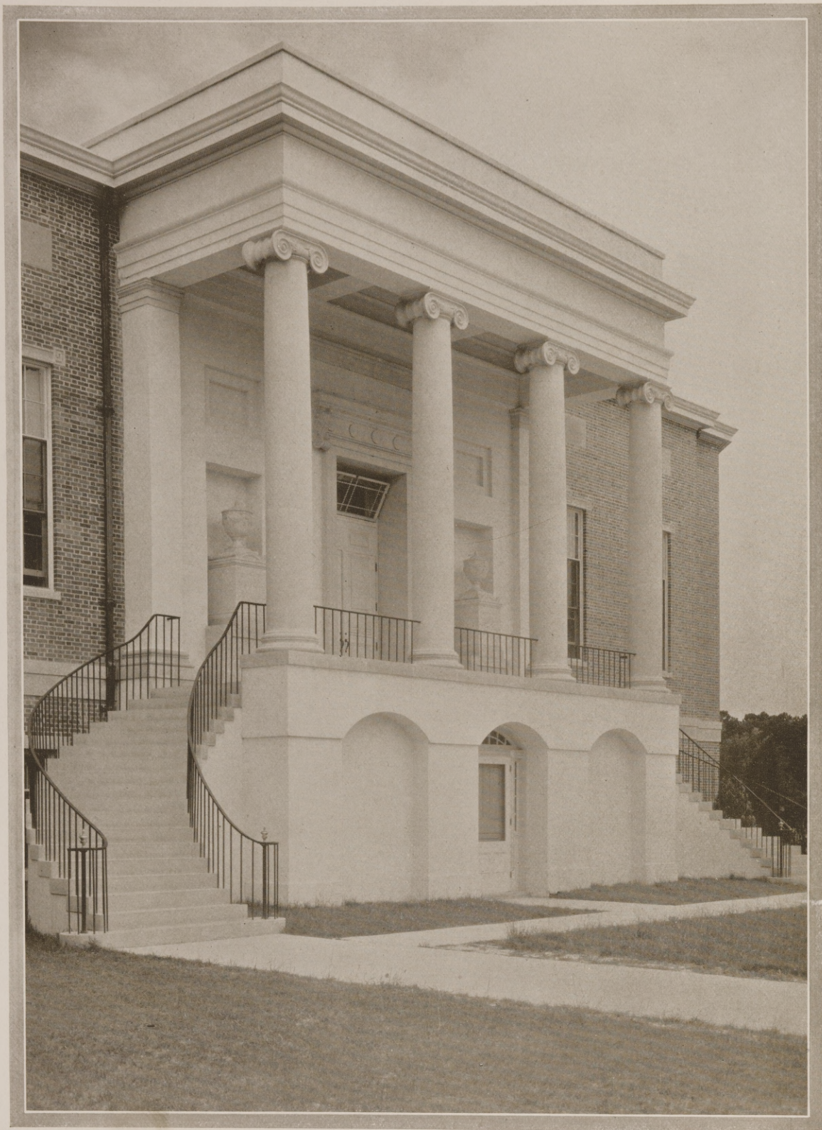
LIBRARY, WESLEYAN COLLEGE, MACON, GA. HENTZ, ADLER & SHUTZE, ARCHITECTS
