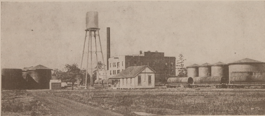
A view of a packing plant where cottonseed oil is taken from the large tanks. Concrete enters largely in construction of these tanks.
