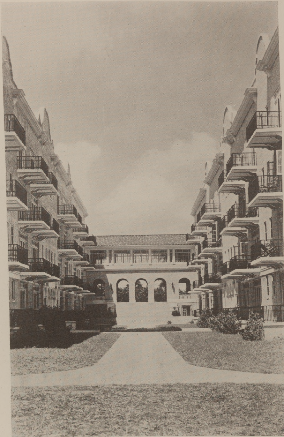
VIEW OF COURT ORANGE COURT APARTMENT, ORLANDO, FLA. G. LLOYD PREACHER, ARCHITECT
