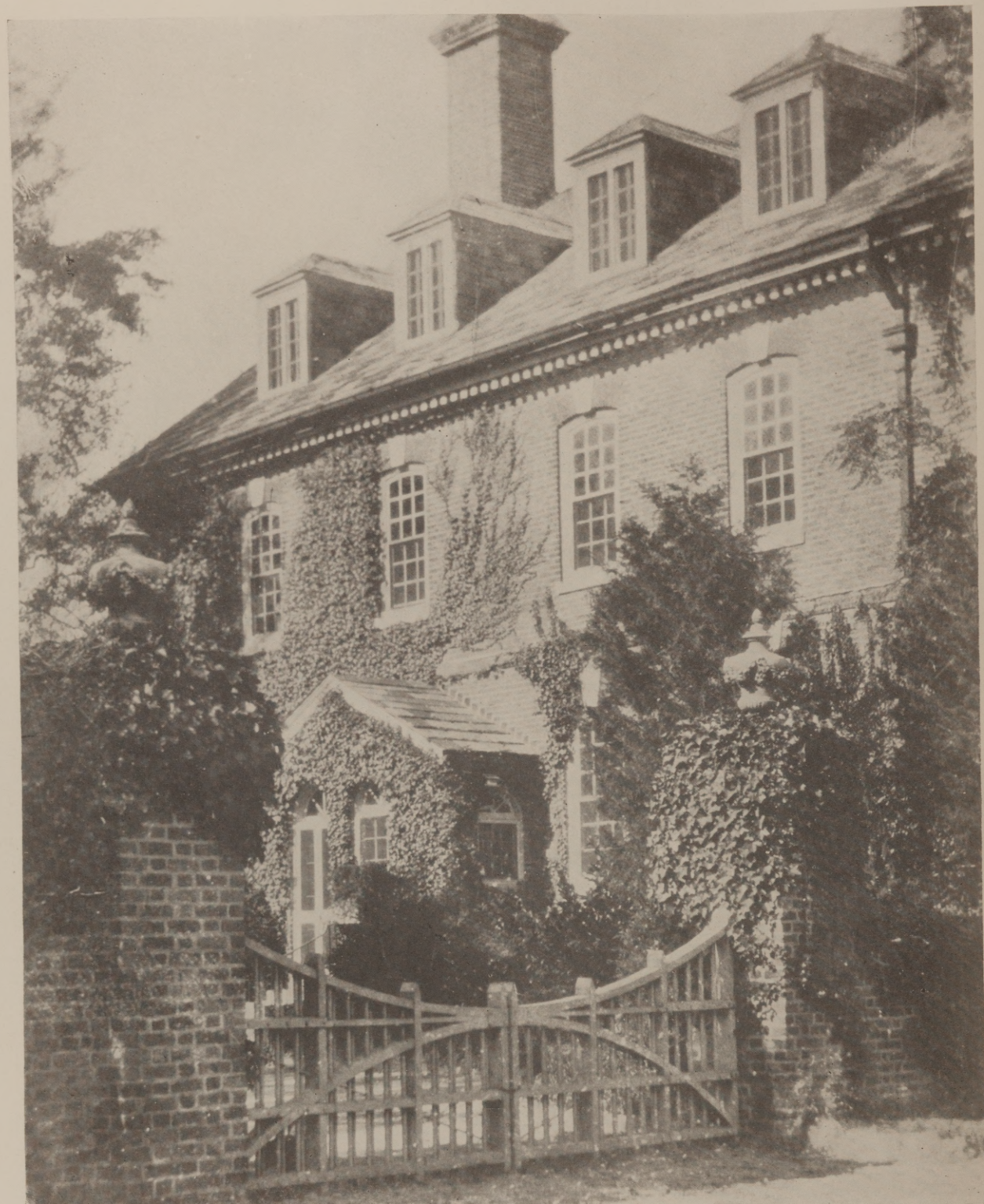
REAR DETAIL NELSON HOUSE, YORKTOWN, VA. BUILT BY THOMAS NELSON, 1740
