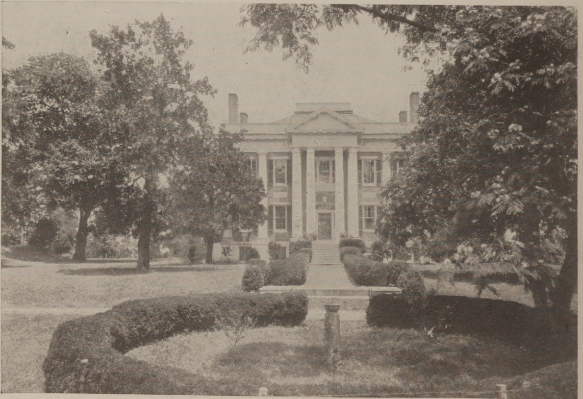
FRONT ELEVATION HAMPSTEAD, NEW KENT COUNTY, VA. BUILT BY CONRAD WEBB, 1820.
