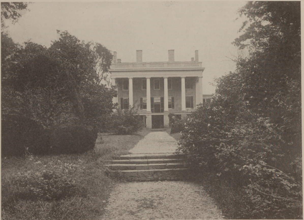
REAR ELEVATION VAN LEW HOUSE, RICHMOND, VA. BUILT BY JNO. ADAMS. ABOUT 1790
