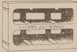
Bottom View of McIntyre Building Tile
