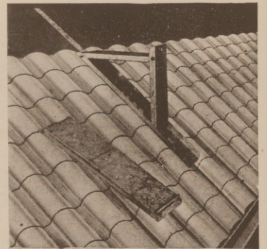
Spanish Tile Roof.
