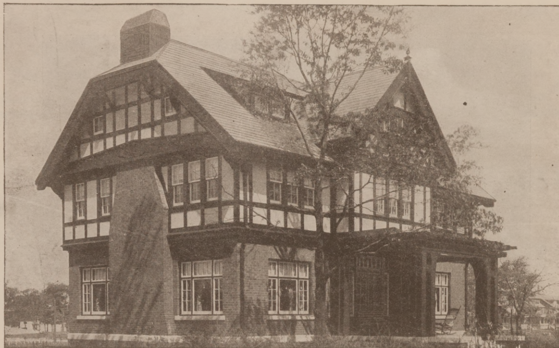
Roof covered with Ambler Asbestos Shingles (Century Brand)—American method. Upper sidewalls covered with Ambler Asbestos Building Lumber—Half-timber effect.
