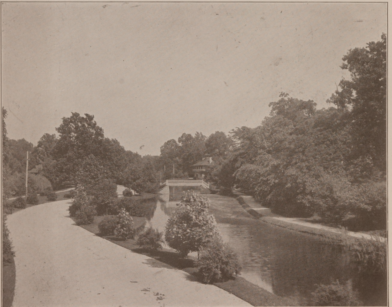
Park Stream Protected by Concrete Embankments.
