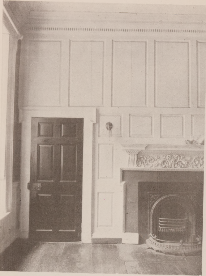
The dining room is paneled on the fireplace side. Note the detail in the mantel and the simple but effective paneling, also the wide pine boards in the floor.
