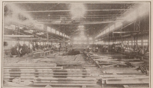
INTERIOR VIEW OF OUR STRUCTURAL STEEL PLANT.
