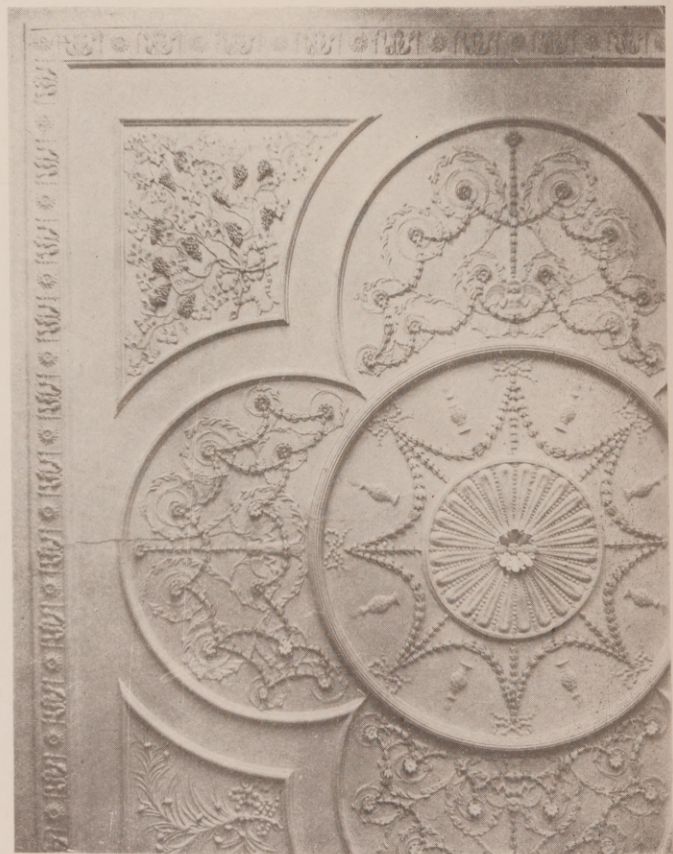
Detail of ceiling panel.
