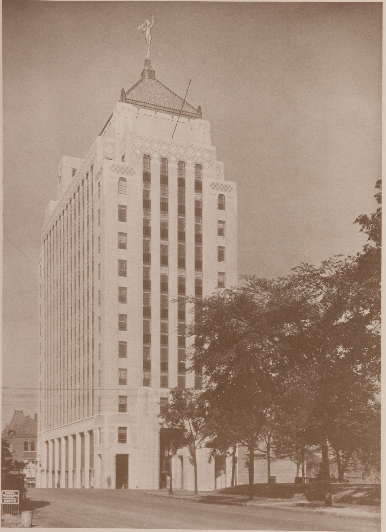
ALABAMA POWER CO. BLDG., BIRMINGHAM, ALA. WARREN, KNIGHT & DAVIS, ARCHITECTS
