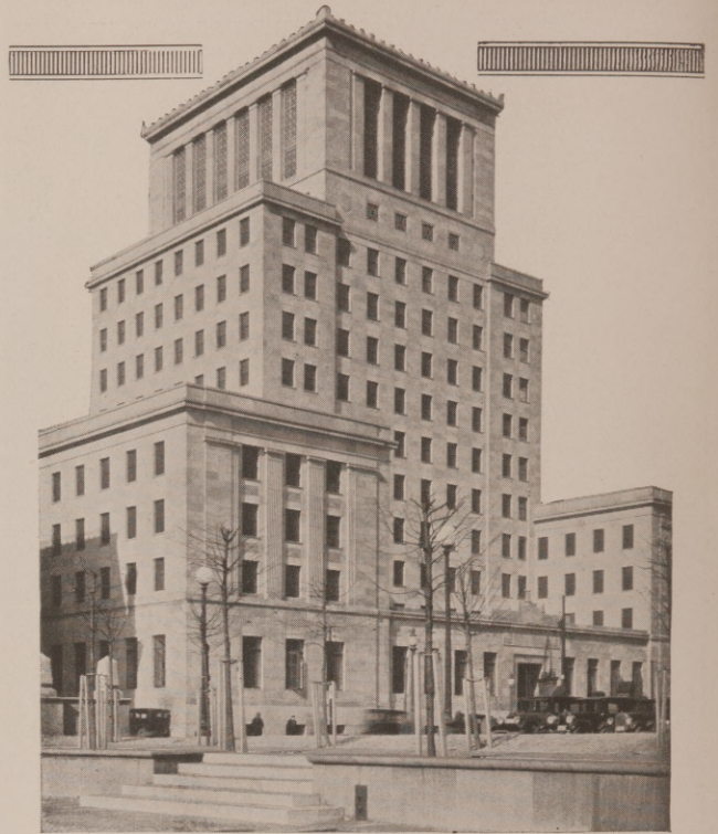
MUNICIPAL BUILDING BALTIMORE, MD.
