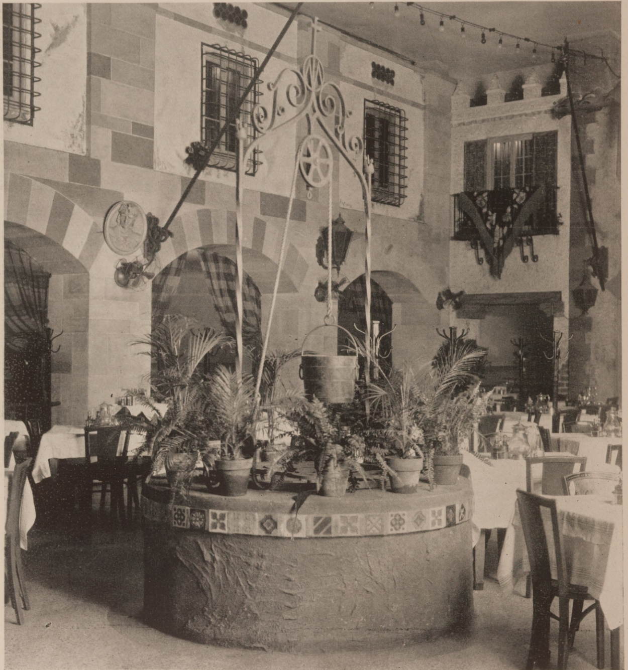
Detail of Old Well Head in Morrison Cafeteria, New Orleans, La.
