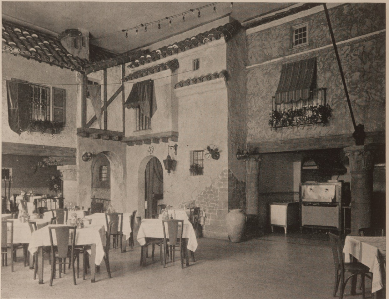
END DETAIL, MORRISON CAFETERIA, NEW ORLEANS, LA. FAVROT & LIVAUDAIS, ARCHITECTS
