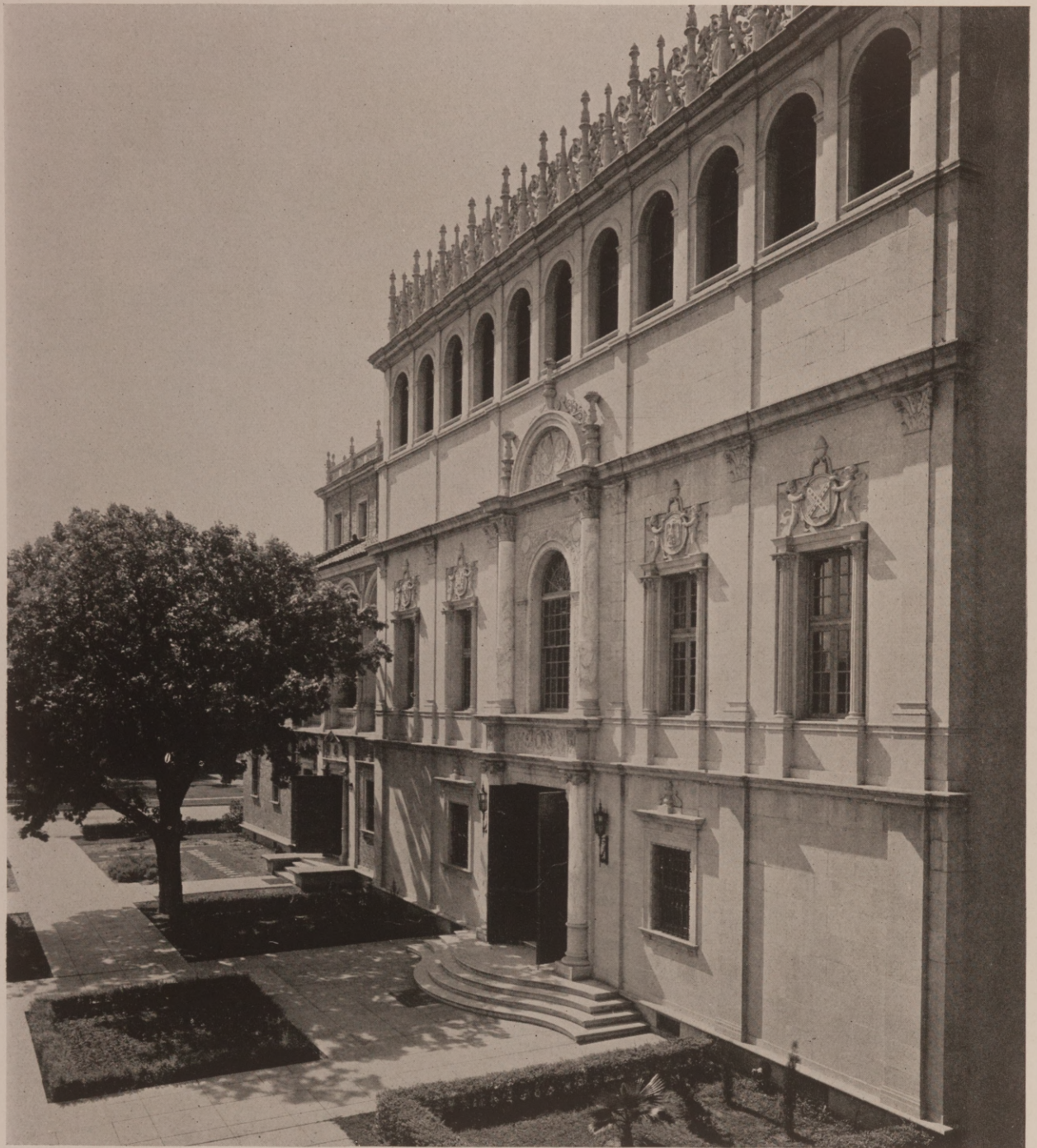
ENTRANCE DETAIL, HOUSTON PUBLIC LIBRARY, HOUSTON, TEXAS
