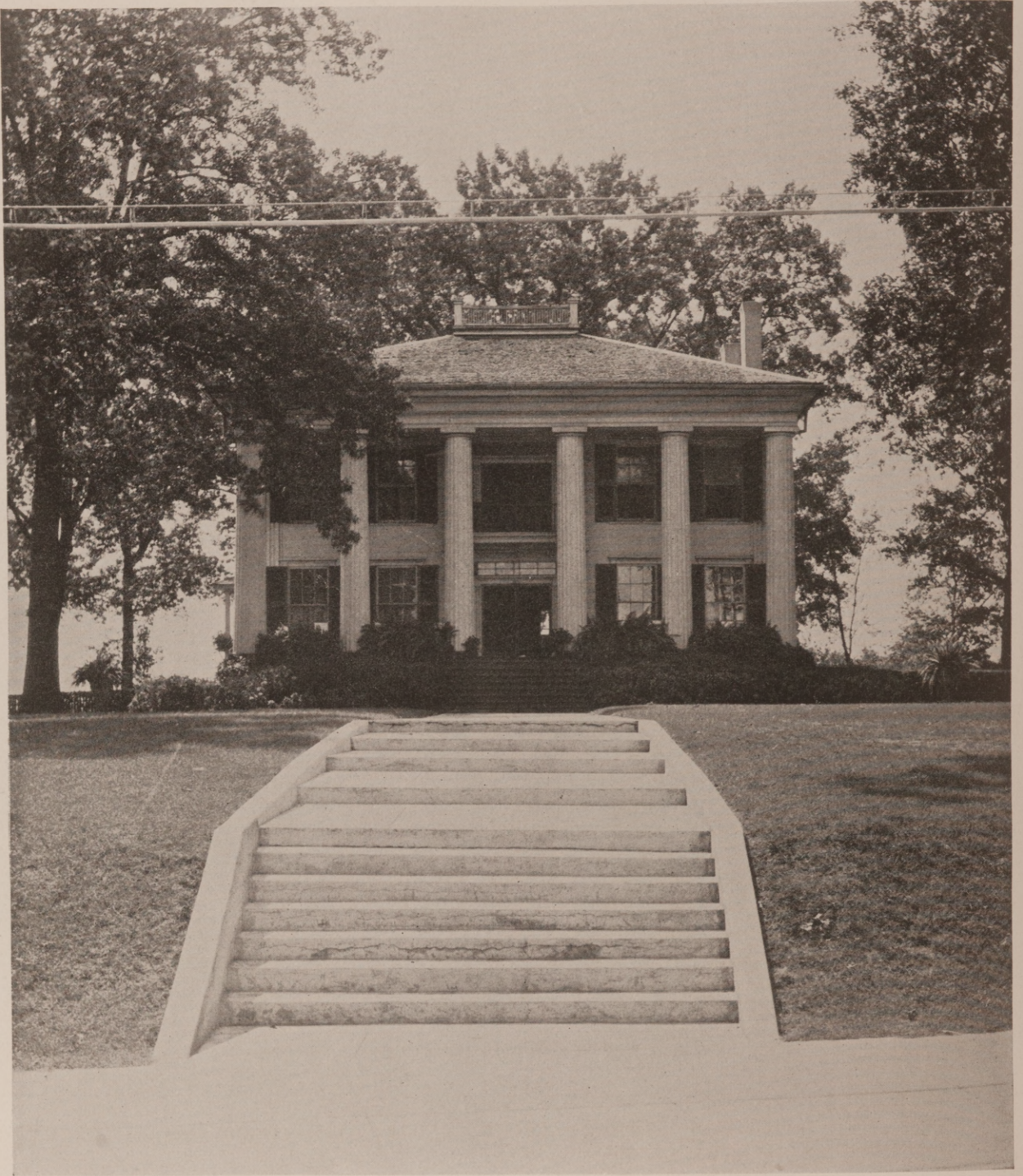
DODD HOUSE, LAGRANGE, GA. BUILT 1845
