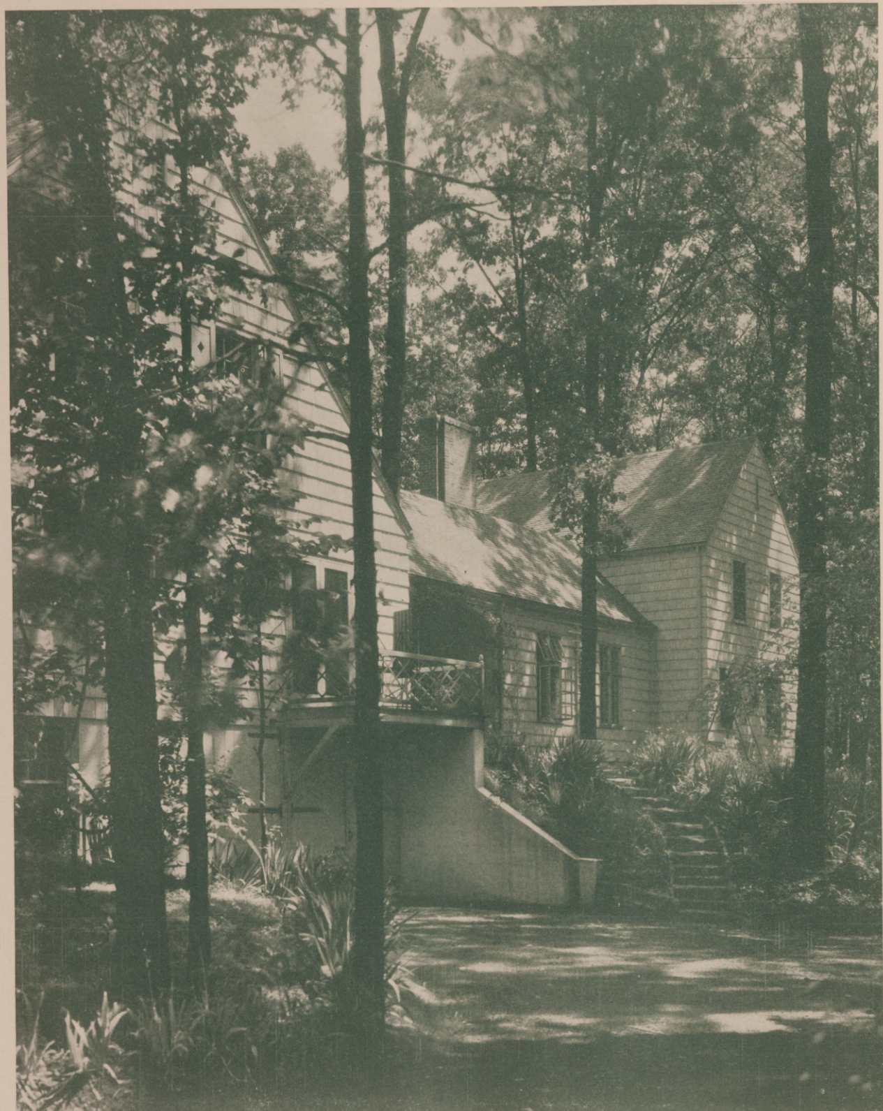
TERRACE SIDE THE YEAGER-McDOWELL HOUSE, KNOXVILLE, TENN. BARBER & McMURRAY, ARCHITECTS
