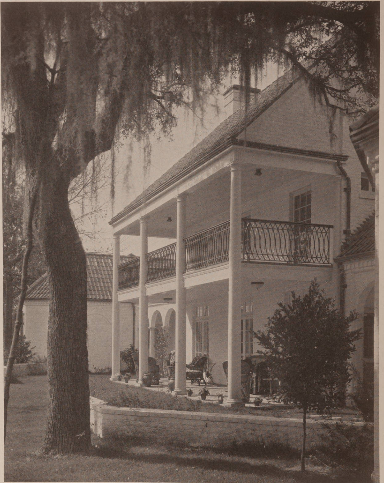
HOUSE OF C. N. MASON, YEOMANS HALL, CHARLESTON, S. C. FRANKLIN ABBOTT, ARCHITECT
