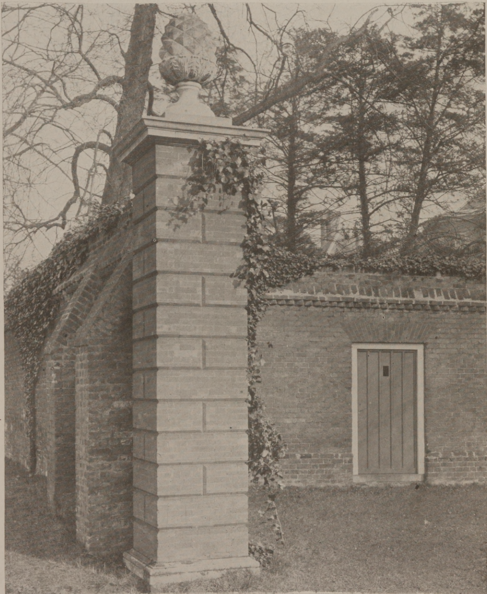
GARDEN WALL PIER, HAM HOUSE, SURREY Built about 1780, of "glowing" red rubbers with V-shaped rustication carefully chiseled out.
