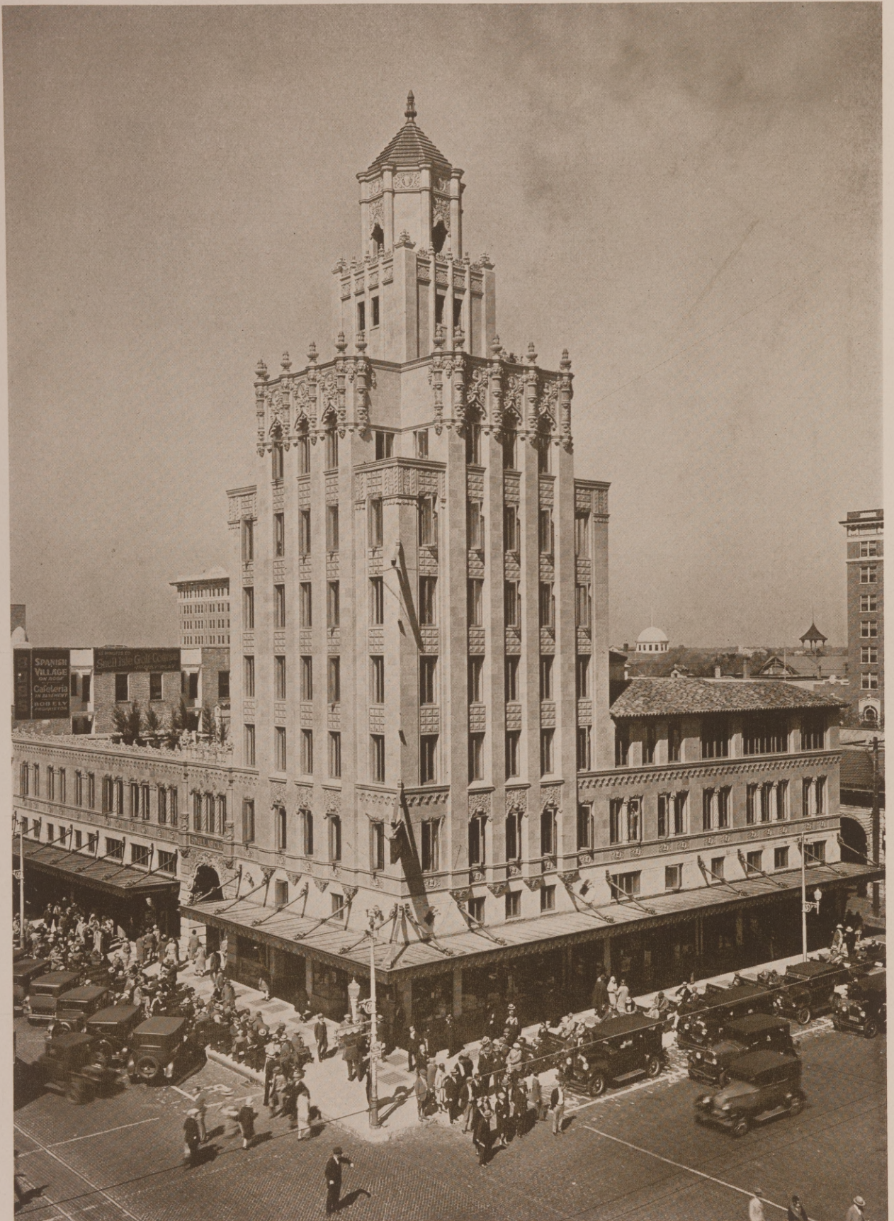
SNELL ARCADE BUILDING, ST. PETERSBURG, FLA. KIEHNEL & ELLIOTT, ARCHITECTS
