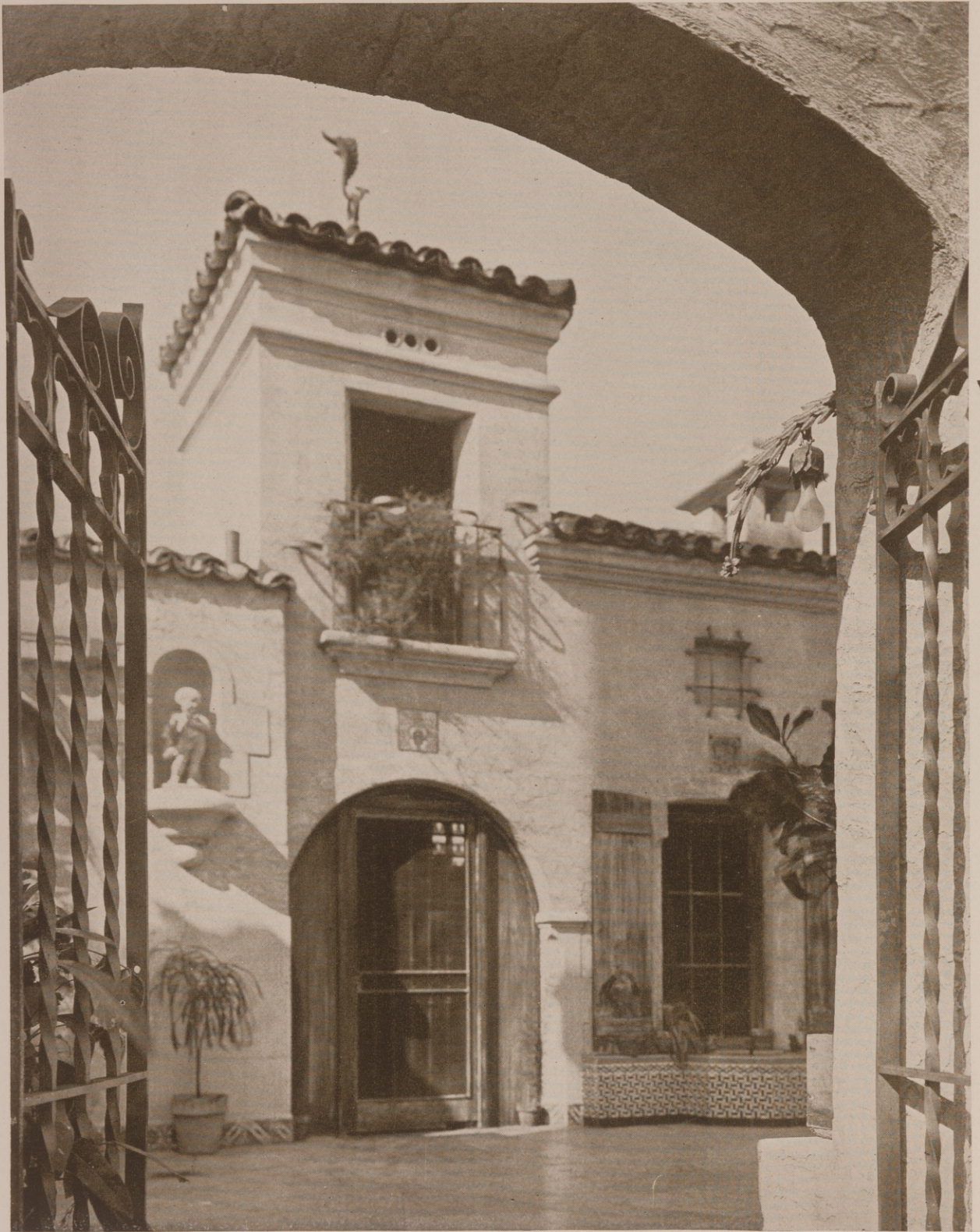
DETAIL ON ROOF GARDEN SNELL ARCADE BUILDING, ST. PETERSBURG, FLA. KIEHNEL & ELLIOTT, ARCHITECTS
