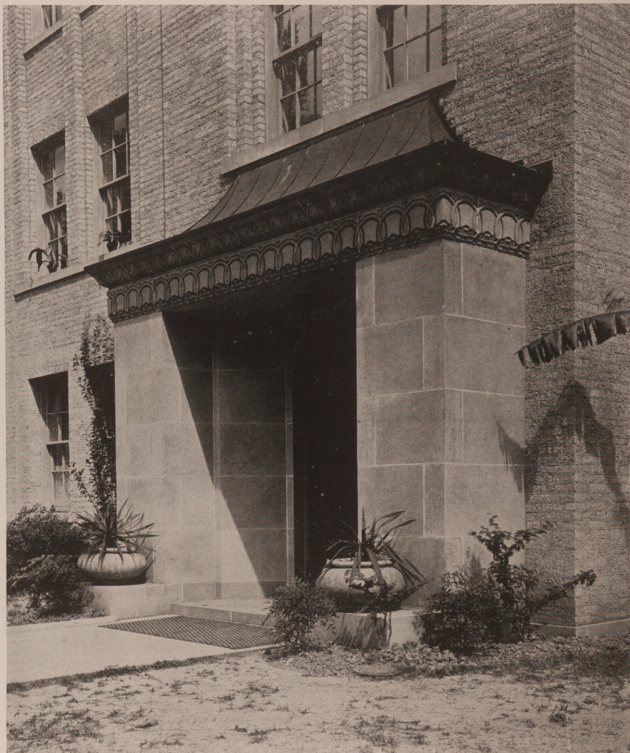
ENTRANCE DETAIL TO SUNDAY SCHOOL ROOMS, TEMPLE SINAI, NEW ORLEANS, LA.
