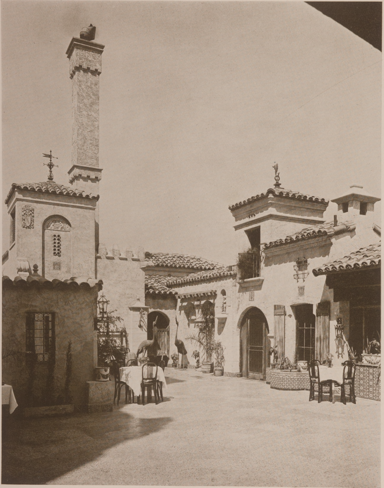
DETAIL ON ROOF GARDEN SNELL ARCADE BUILDING, ST. PETERSBURG, FLA. KIEHNEL & ELLIOTT, ARCHITECTS
