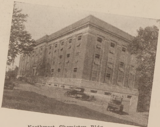
Northwest Chemistry Bldg., Bureau of Standards, Washington, D. C.
