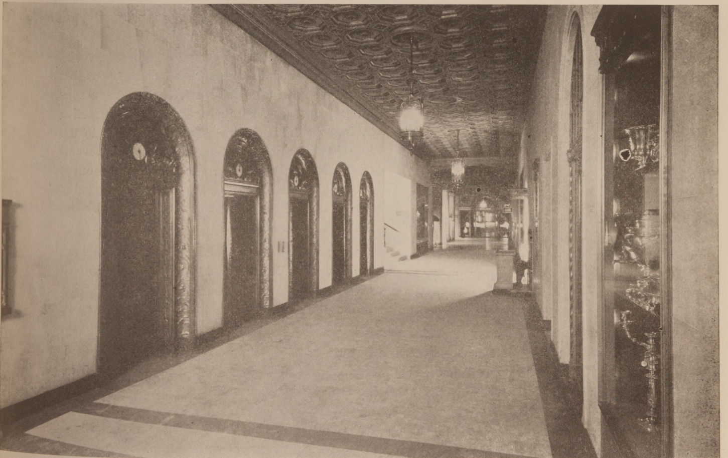
PART OF FRONT LOBBY—THE BULKLEY BUILDING, CLEVELAND, OHIO. C. HOWARD CRANE, ARCHITECT.
