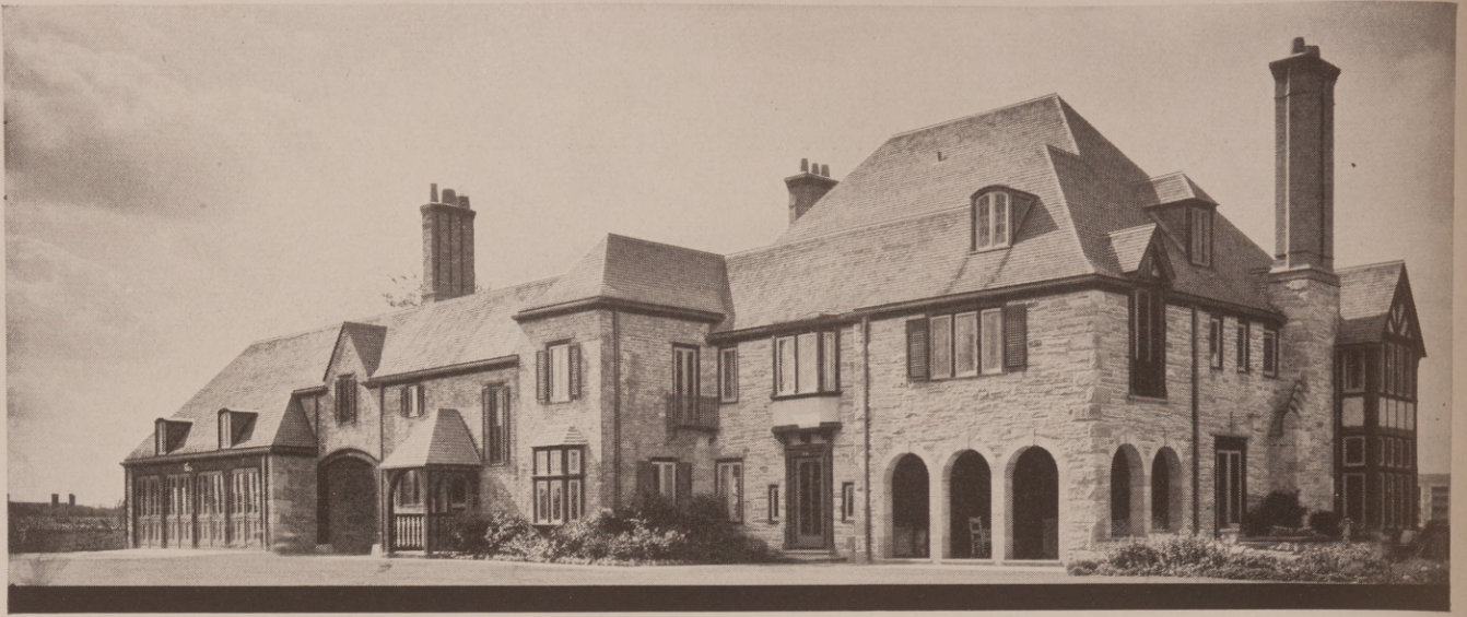
Built-in conduit and nine outlets provide for telephone convenience in the residence of Mr. Wilbert J. Austin, Sberbrooke Road, Shaker Heights, Cleveland, Ohio. MAIER & WALSH, Architects, Cleveland
