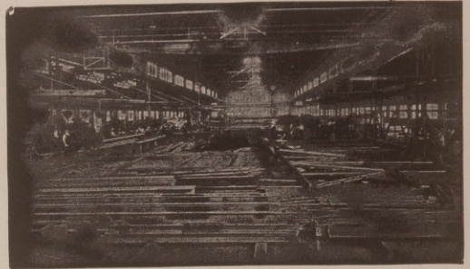
INTERIOR VIEW OF OUR STRUCTURAL STEEL PLANT
