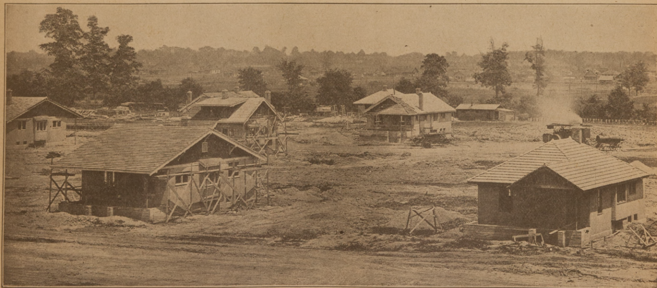
Houses for Lafayette Motors Employees. Roofed with Concretile. J. Edwin Kopf, Architects.
