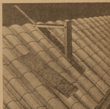
Spanish Tile Roof.
