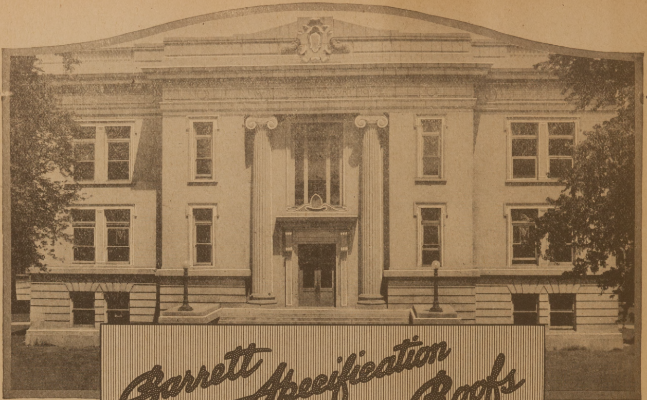
20 Year Barrett Specification Bonded Roof on Marion County Court House, Salem, Ill.
