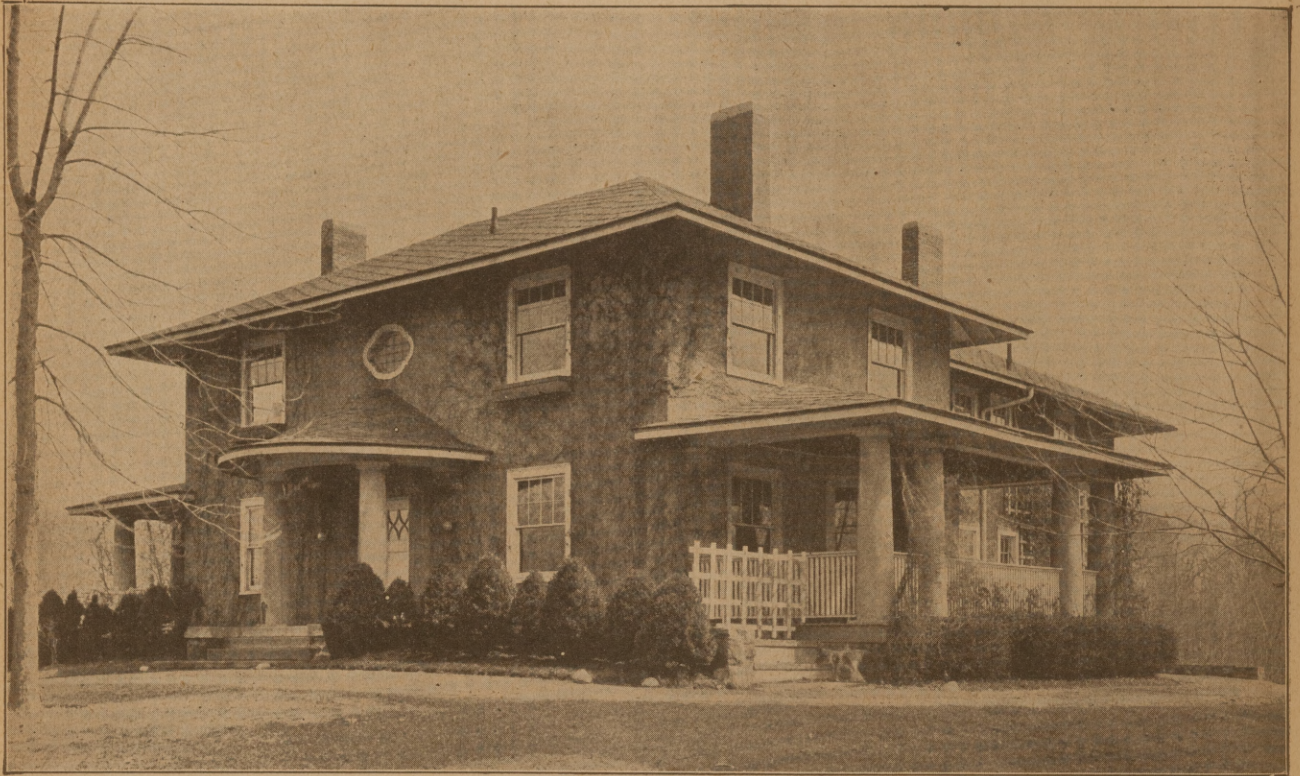
Radiant Shingles over old wood shingles.
