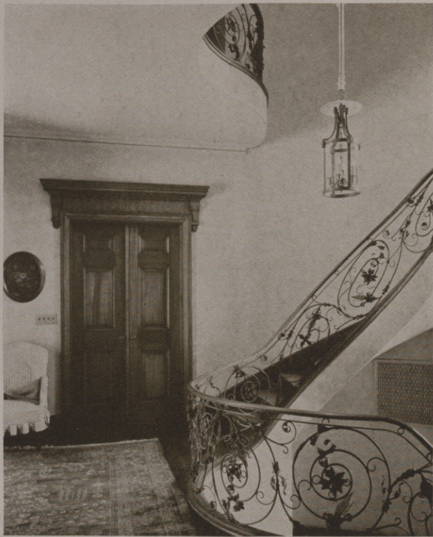
DETAIL OF STAIR
