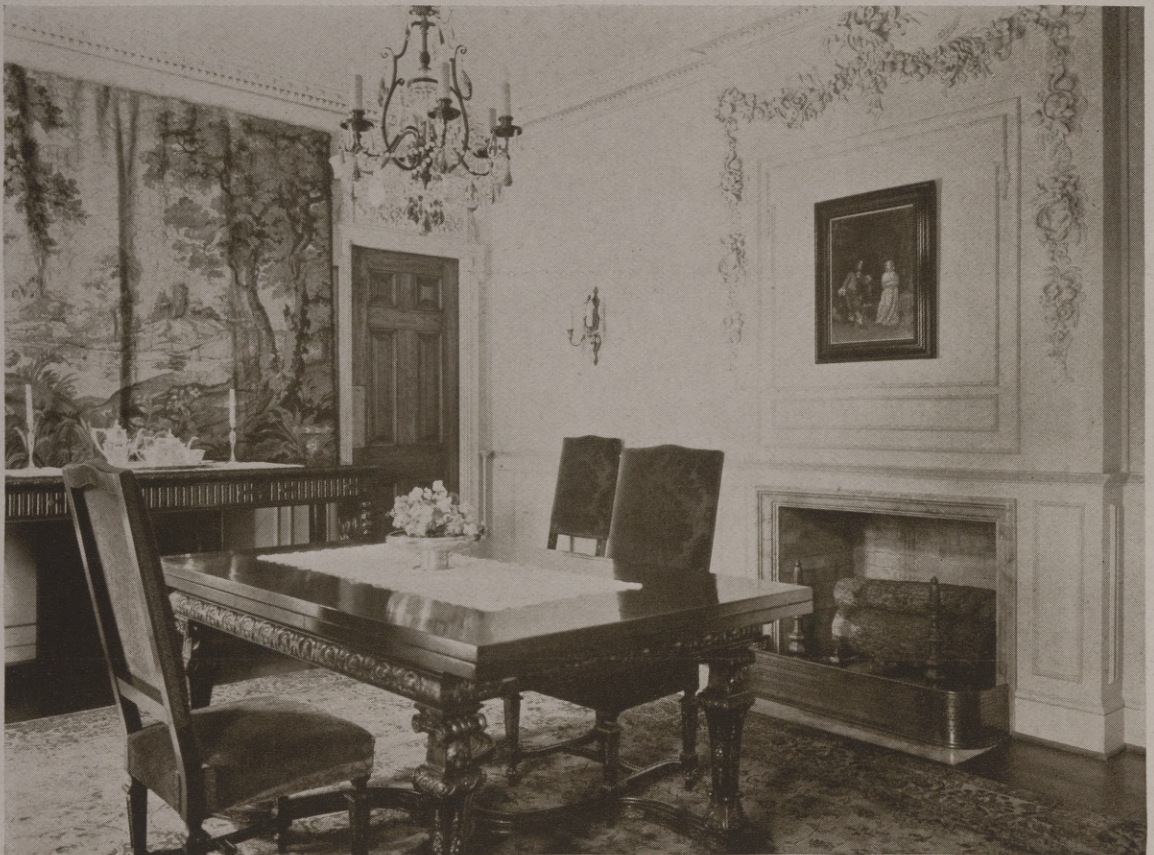
DINING ROOM, HOUSE OF CATOR WOOLFORD, ESQ., ATLANTA, GA. OWEN JAMES SOUTHWELL, ARCHITECT
