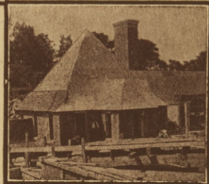
The New British Embassy Building, Washington, D. C. Sir E. L. Lutyens, R. A., Architect, Frederick H. Brooke, Associate Architect. Nailcrete used as structural roof slab--also as nailing base for wood floors. Insert shows application of Nailcrete on roof.
