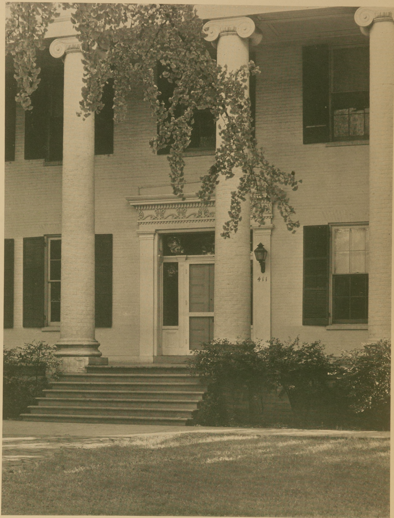
ENTRANCE FRONT THE ALBERT PIKE HOUSE, LITTLE ROCK, ARK. BUILT IN 1840
