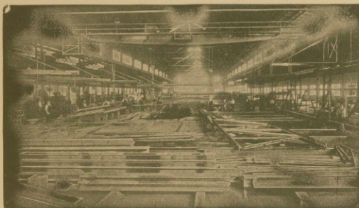
INTERIOR VIEW OF OUR STRUCTURAL STEEL PLANT
