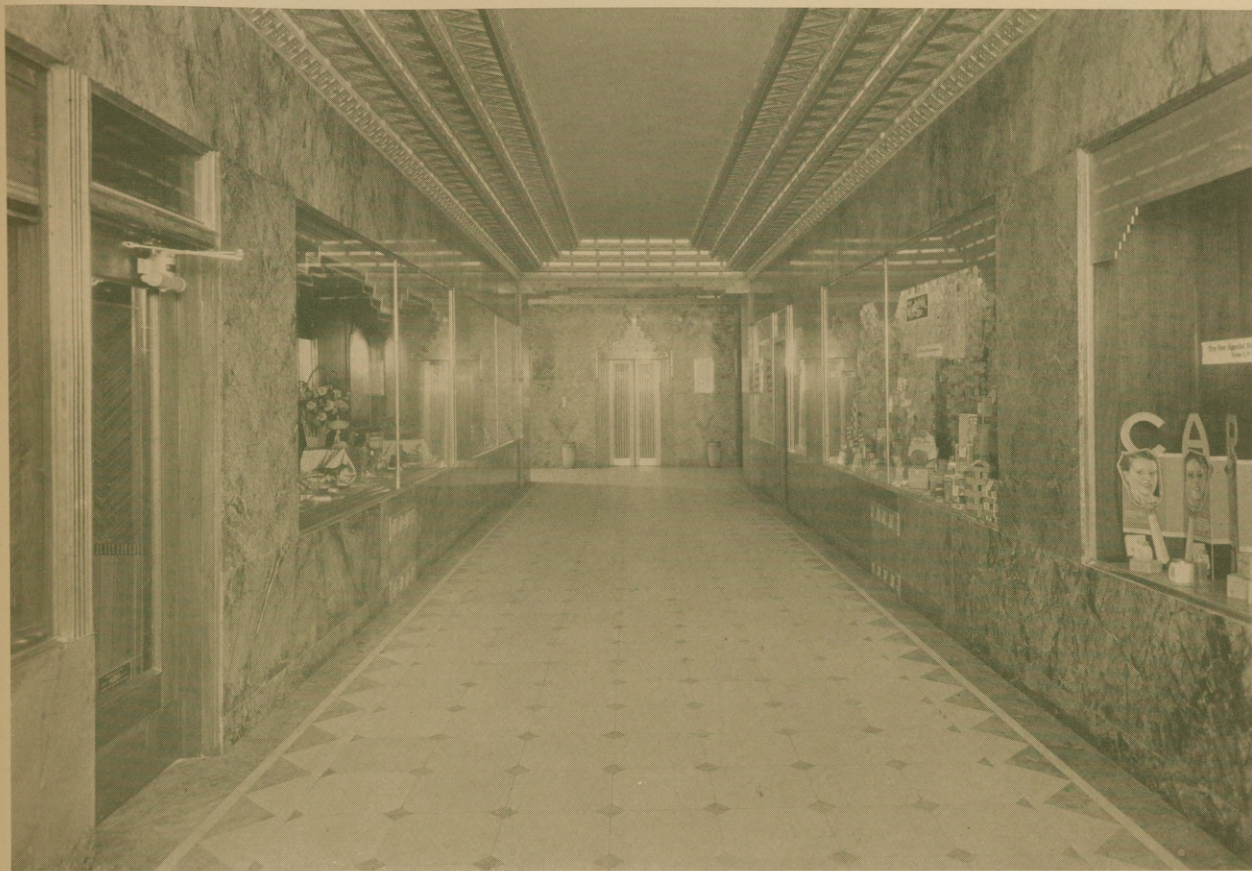
Lobby, Sinclair Building, Fort Worth, Texas
