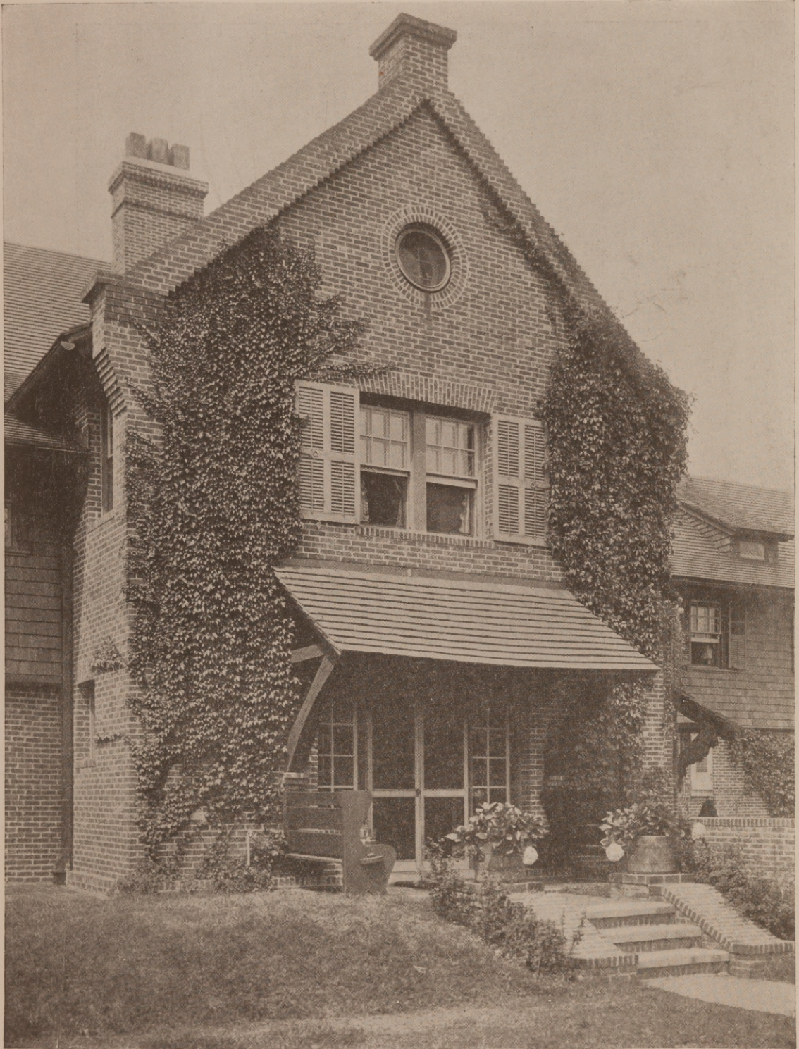
Detail of Residence, Huntington, L. I. Wilson Eyre, Architect
