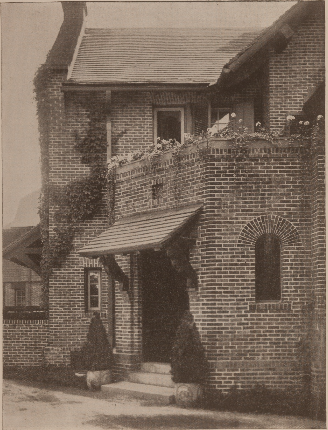
Detail of Residence, Huntington, L. I. Wilson Eyre, Architect Around the corner is this intimate and covered entrance into the main wing of the house. The arched opening lights the vestibule, which is lined with brick.
