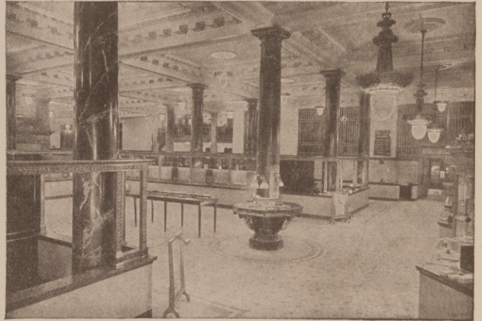
Remodeled fixture with one 300-watt Mazda Lamp and three 40-watt bulbs—420 watts—four foot-candles.
