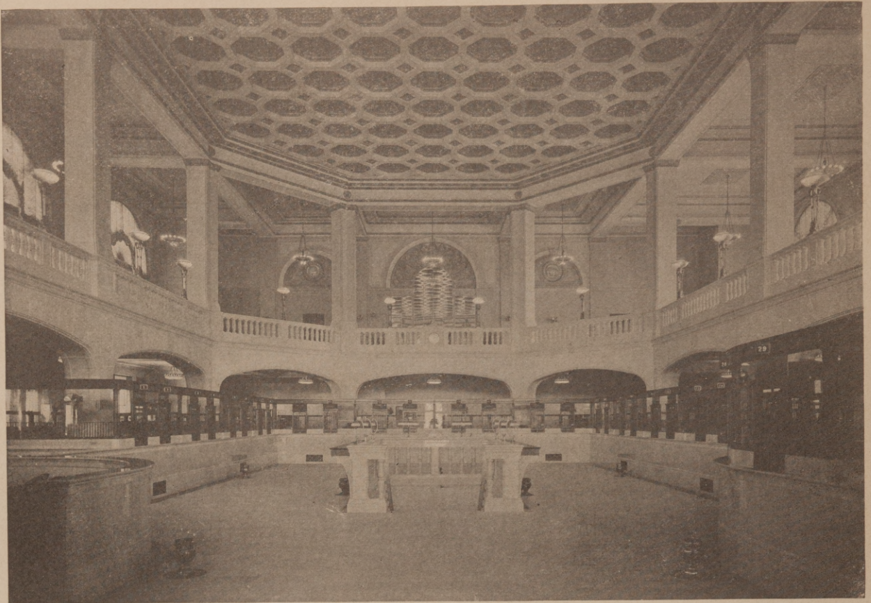
MAIN BANKING ROOM
