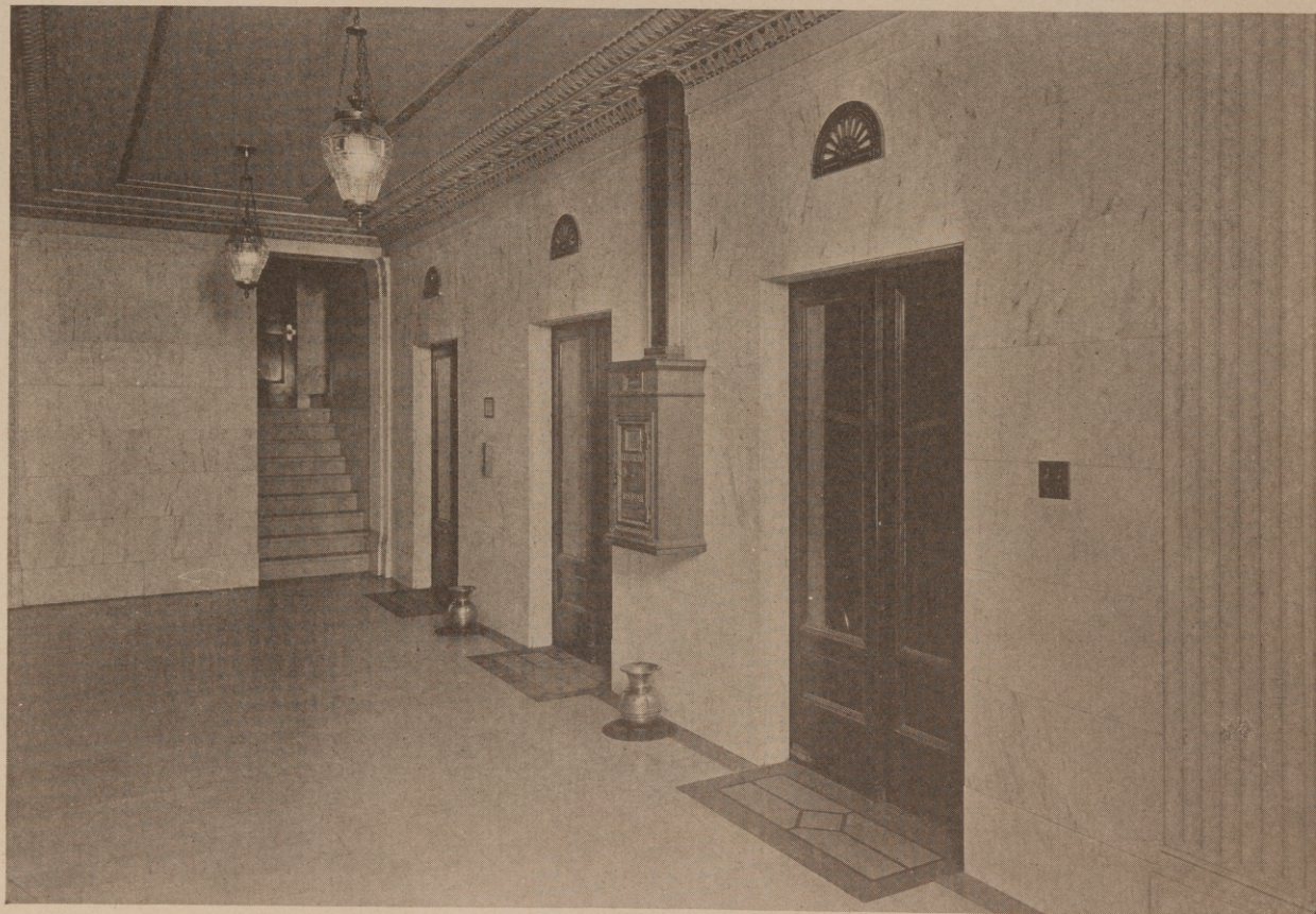
ELEVATOR LOBBY THE FROST NATIONAL BANK, FORT WORTH, TEXAS. SANGUINETT, STAATS & HEDRICK, ARCHITECTS.
