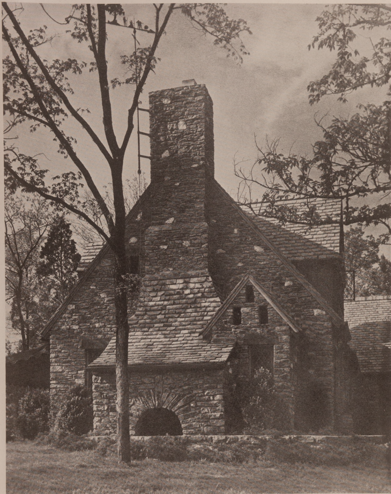
HOUSE OF NEWMAN CHEEK, ESQ., NASHVILLE, TENN. WELBY PUGIN, ARCHITECT
