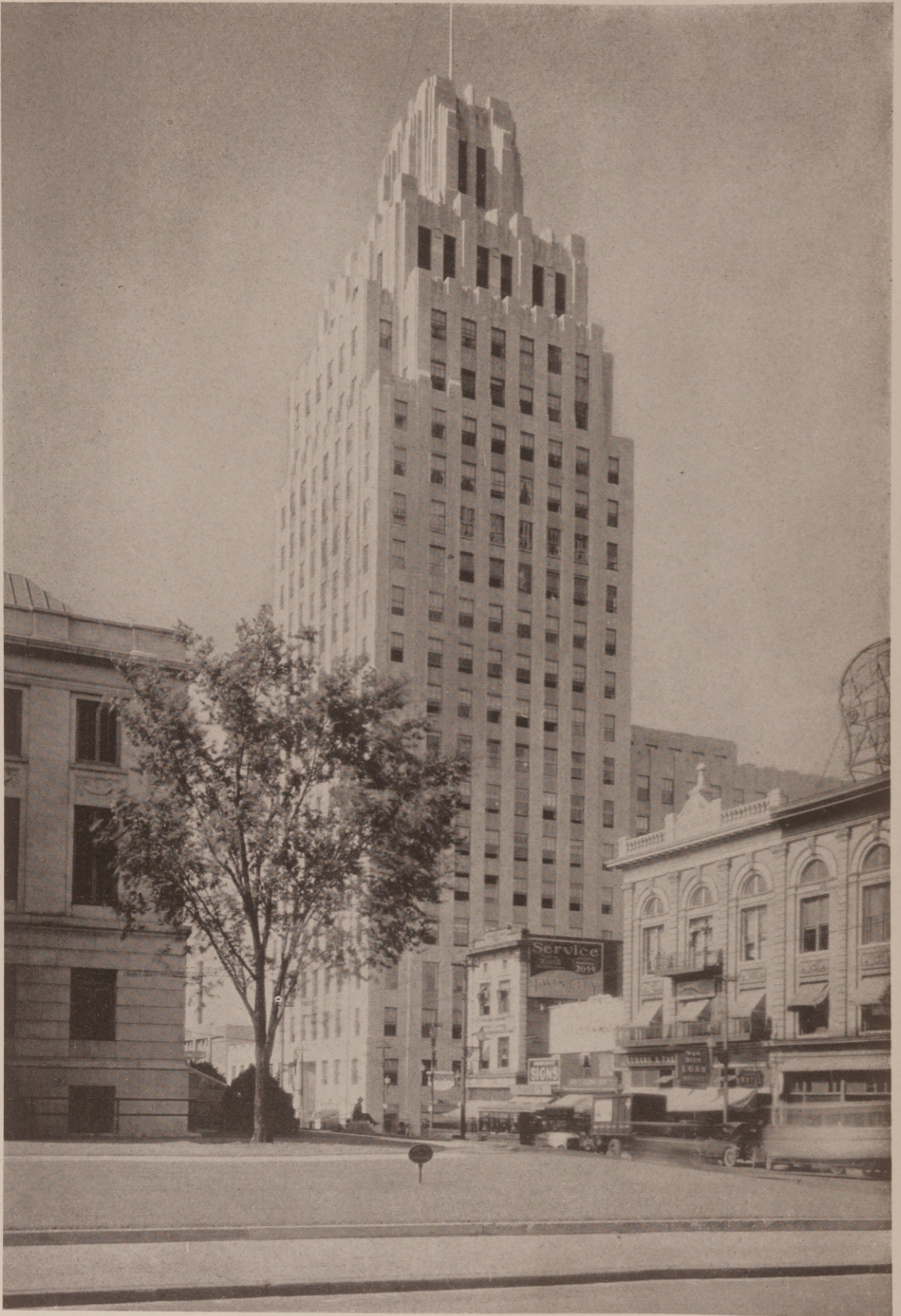
R. J. REYNOLDS TOBACCO COMPANY BUILDING, WINSTON-SALEM, N. C. SHREVE & LAMB, ARCHITECTS
