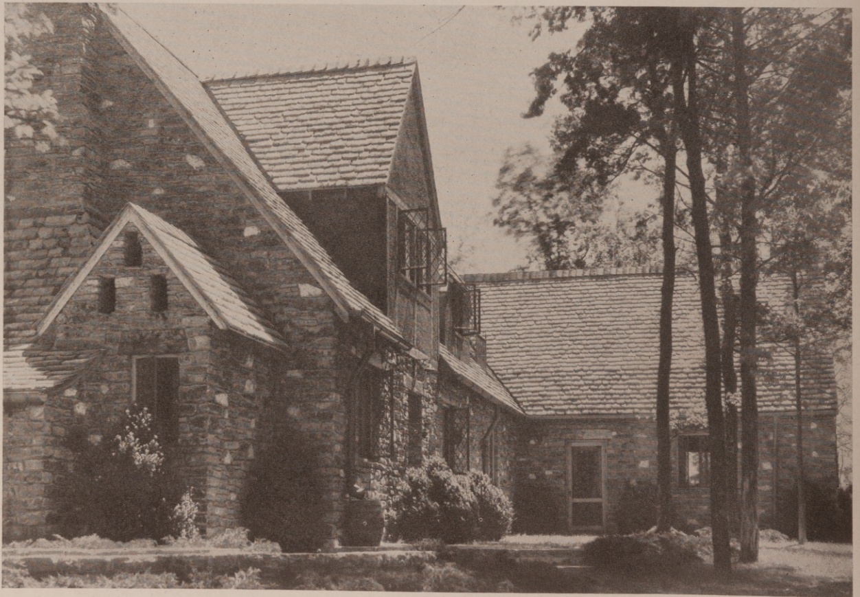
HOUSE OF NEWMAN CHEEK, ESQ., NASHVILLE, TENN. WELBY PUGIN, ARCHITECT
