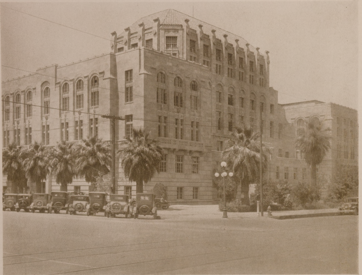
MARICOPA COURT HOUSE AND CITY HALL, PHOENIX, ARIZONA
