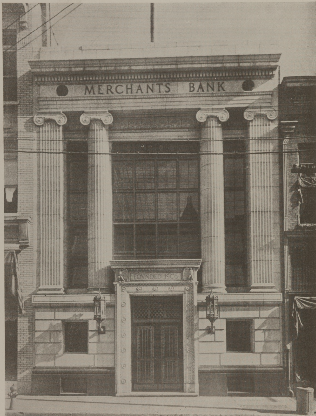
MAIN VIEW MERCHANTS NATIONAL BANK, DURHAM, N. C. ALFRED C. BOSSOM, ARCHITECT
