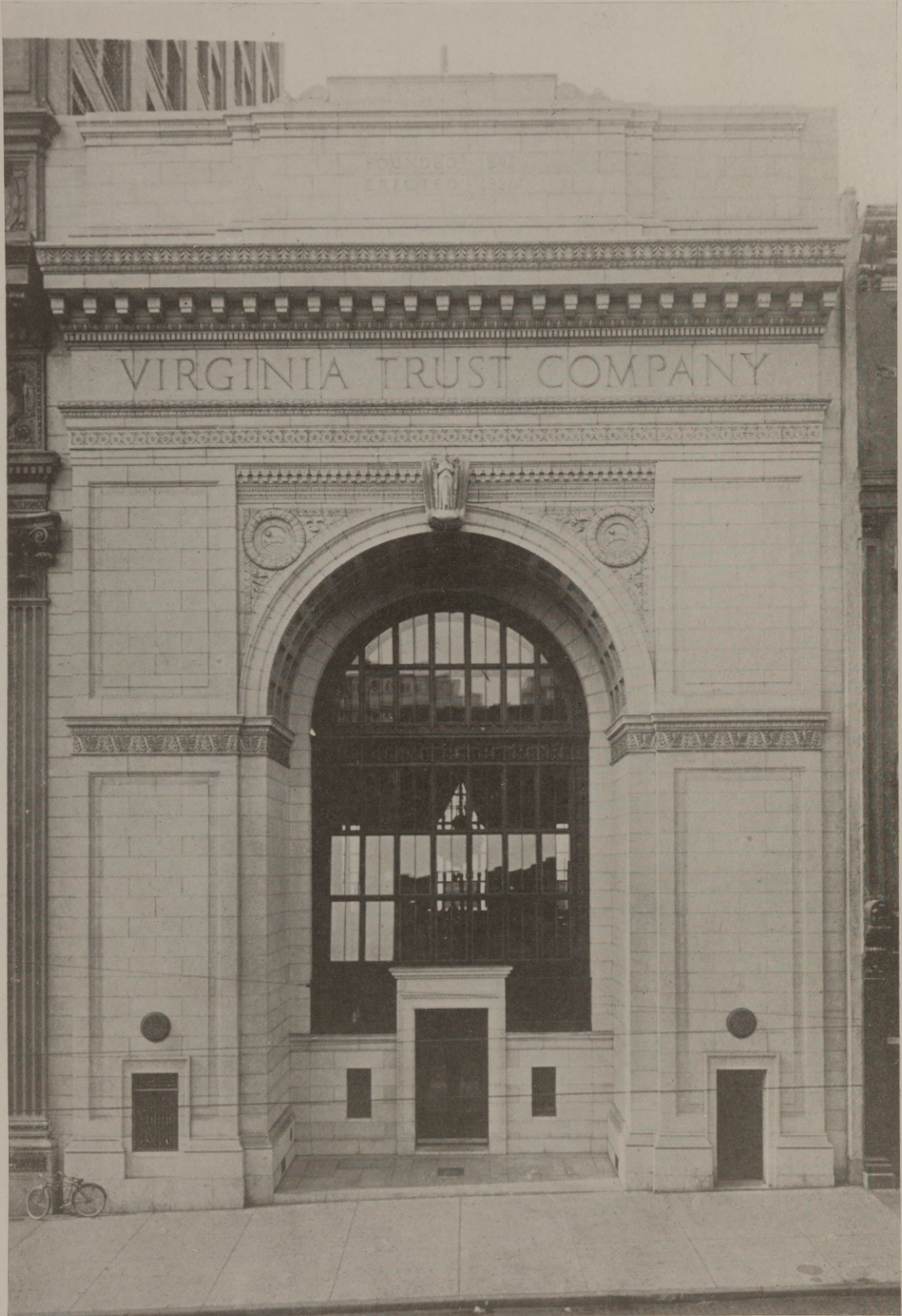
MAIN VIEW VIRGINIA TRUST COMPANY, RICHMOND, VA. ALFRED C. BOSSOM, ARCHITECT
