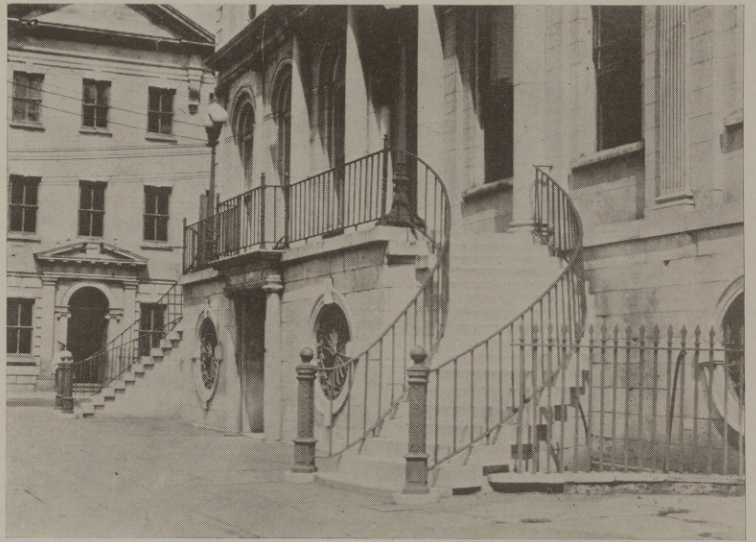
COURTHOUSE (LEFT); CITY HALL (RIGHT).
