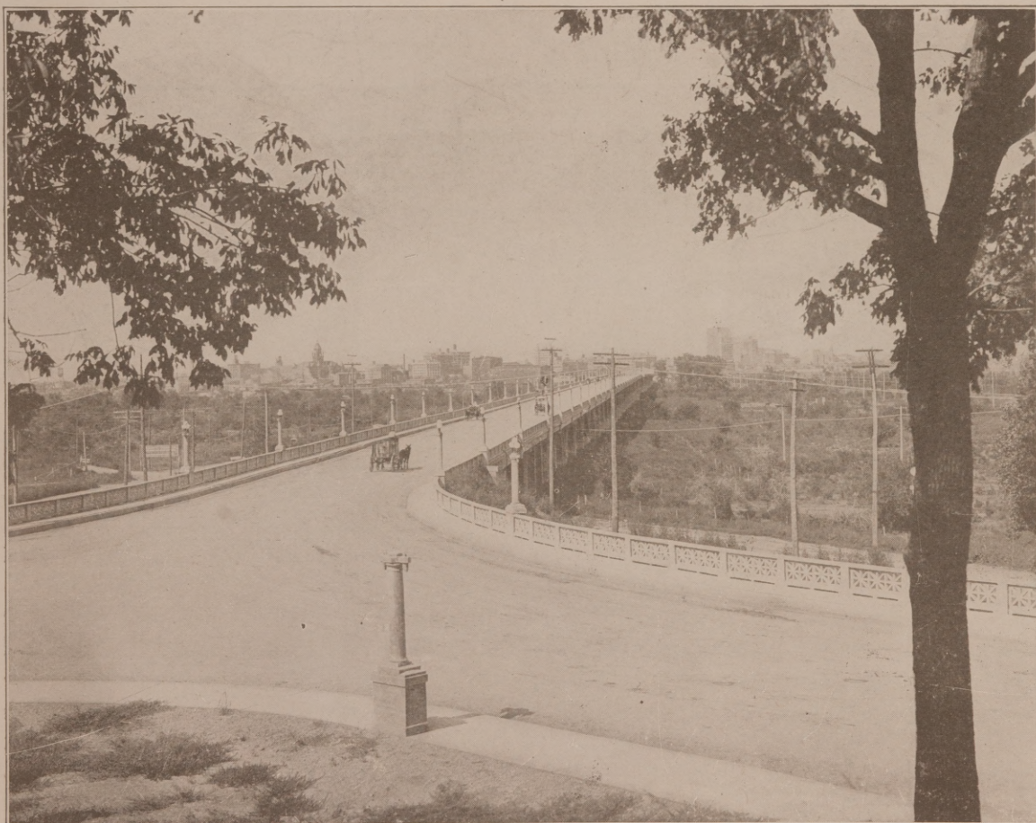
Skyline of Dallas from Oak Cliff End of Viaduct—Longest Concrete Viaduct in World.
