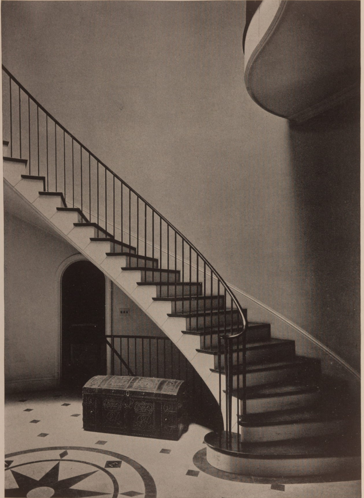
DETAIL STAIRHALL, MIRADOR, GREENWOOD, VIRGINIA DELANO & ALDRICH, ARCHITECTS FOR RESTORATION
