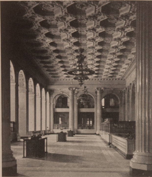
Main Banking Room
