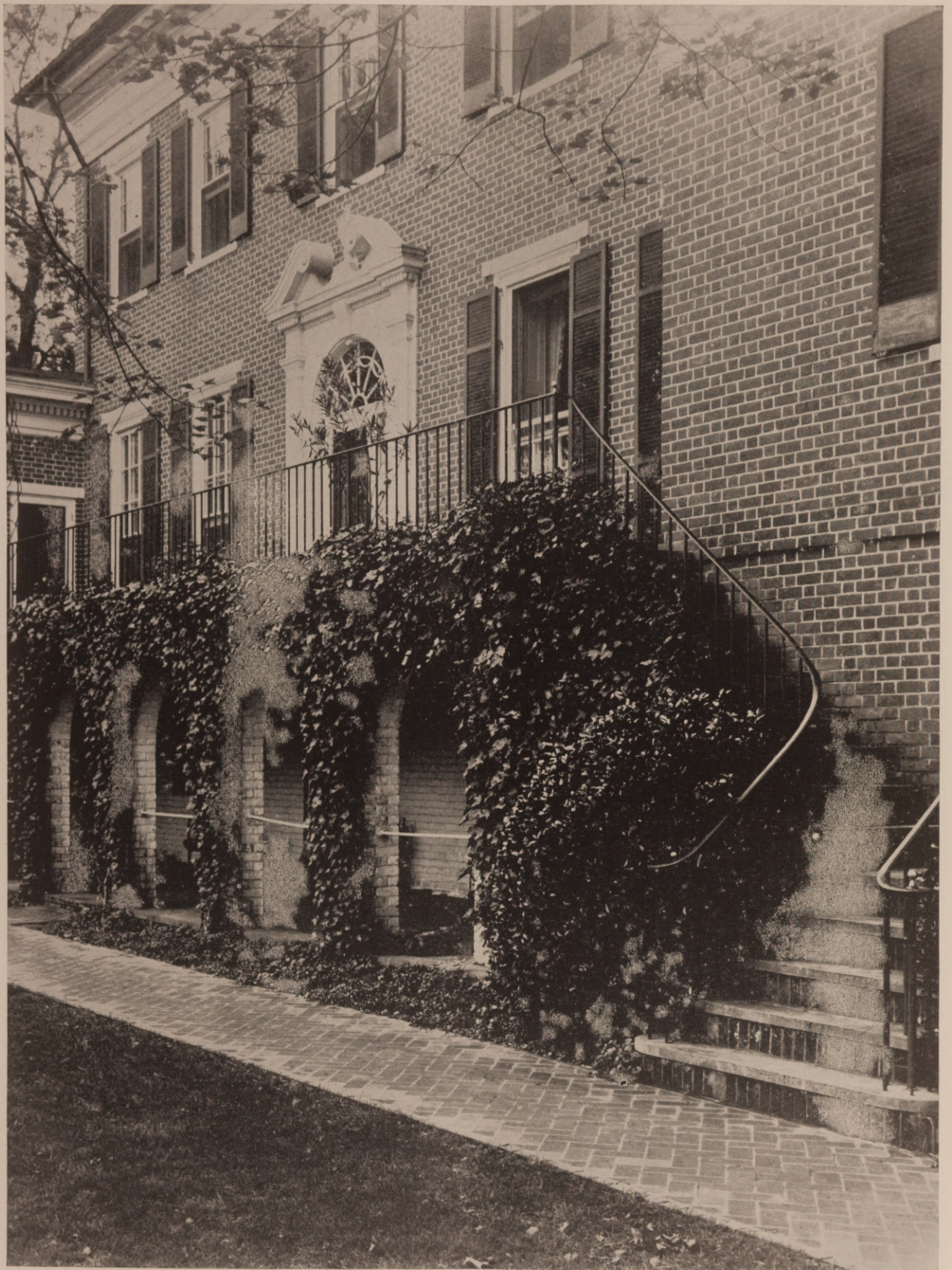
DETAIL GARDEN FACADE, MIRADOR, GREENWOOD, VIRGINIA DELANO & ALDRICH, ARCHITECTS FOR RESTORATION
