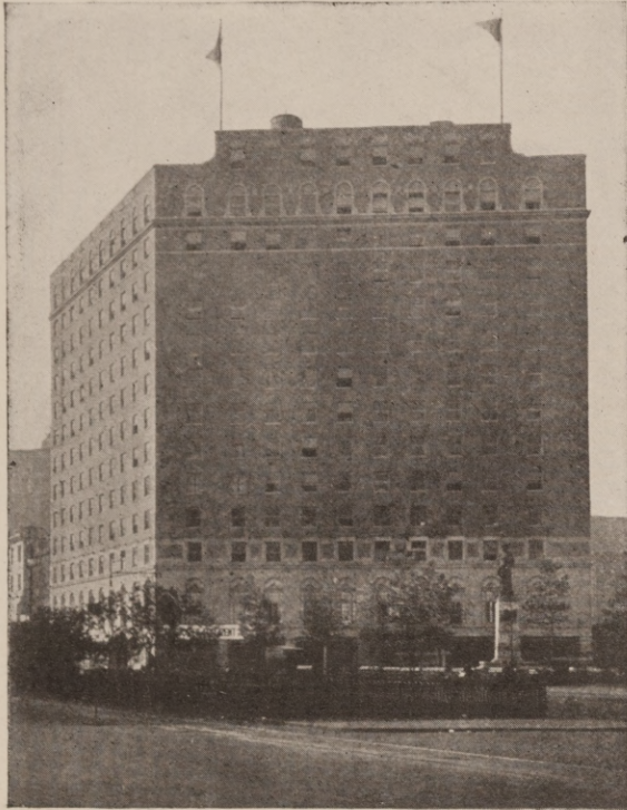
EMPIRE HOTEL, NEW YORK, N. Y. Frederick I. Merrick, Architect
