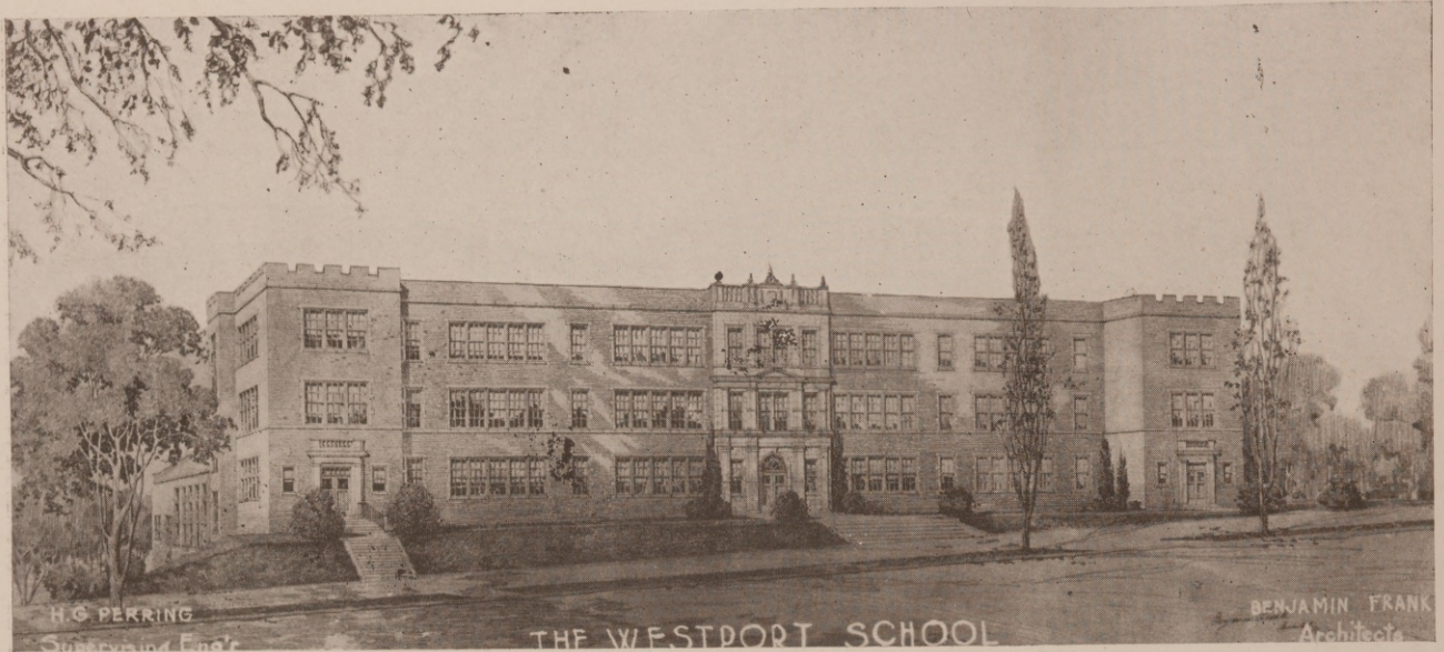
THE WESTPORT SCHOOL, BALTIMORE, MD. BENJAMIN FRANK, ARCHITECT H. G. PERRING, SUPERVISING ARCHITECT
