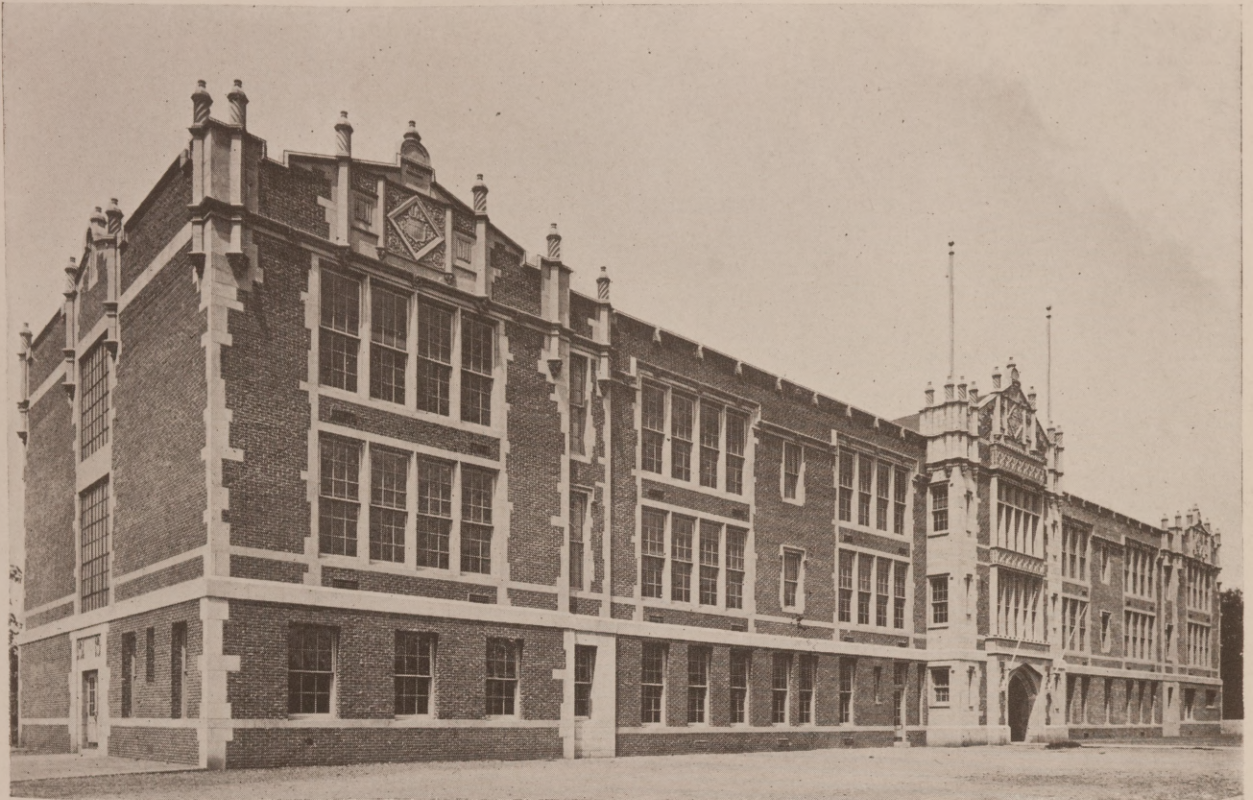
ALEXANDER HAMILTON SCHOOL, BALTIMORE, MD. EDWIN H. GLIDDEN, ARCHITECT H. G. PERRING, SUPERVISING ARCHITECT
