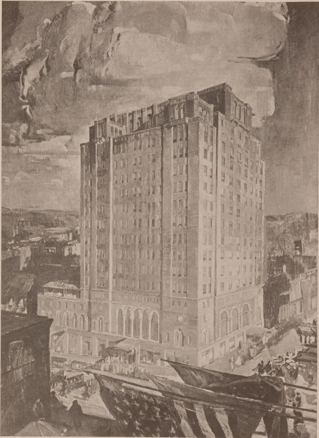
AMERICAN HOTEL—ALLENTOWN, PENNSYLVANIA RITTER AND SHAY, Architects , Philadelphia
