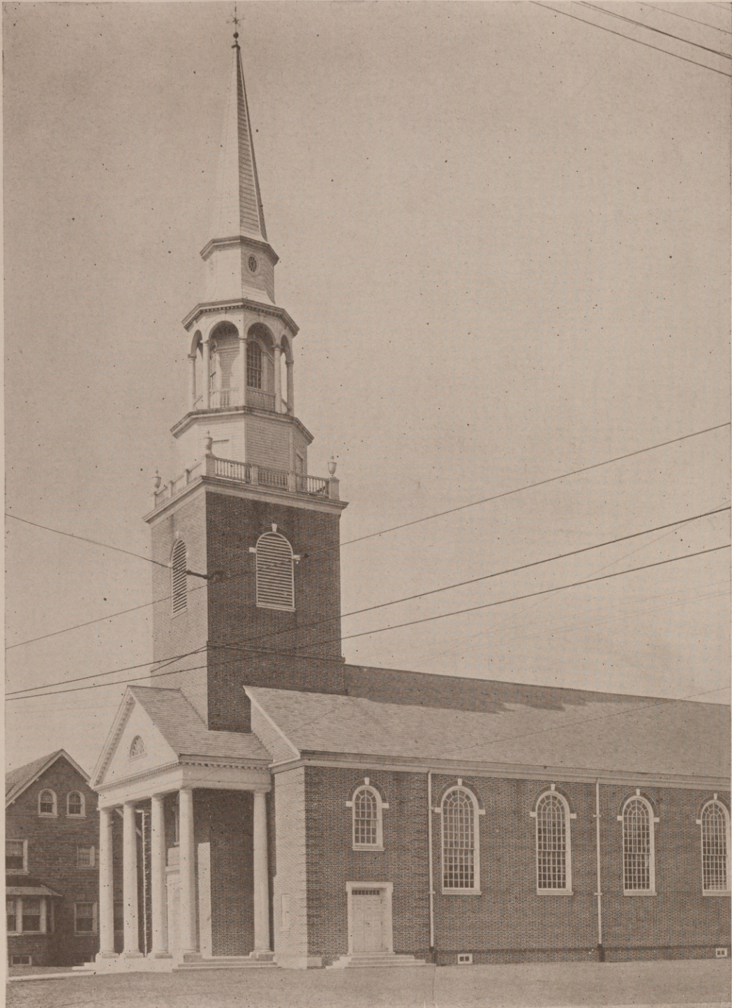
FIRST PRESBYTERIAN CHURCH—CHESTER, PENNSYLVANIA CLARENCE WILSON BRAZER, Architect , Philadelphia FROHNAN AND ROBB, Associates
