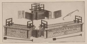
No Buildings to Large, None to Small, to be Built With Them. Build Solid or Double Concrete Walls, So Quickly, So Well. So Reasonable, As to Encourage the Owner to Build Another. Send for Literature
