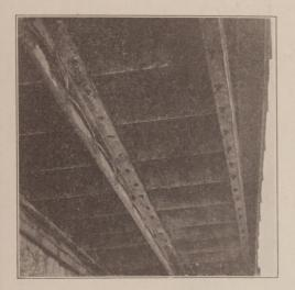
Rust produces an irresistible force when confined between parts.
