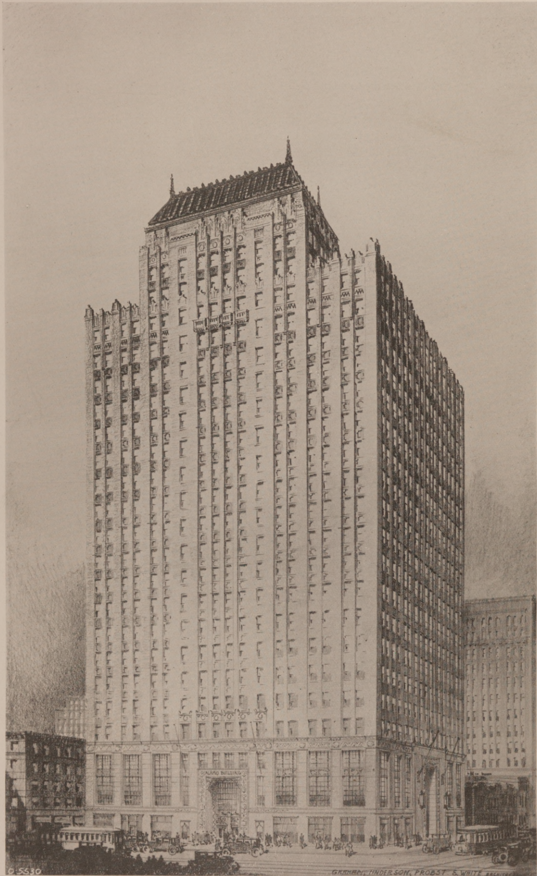
ALAMO NATIONAL BANK, SAN ANTONIO, TEXAS GRAHAM, ANDERSON, PROBST & WHITE, ARCHITECTS
