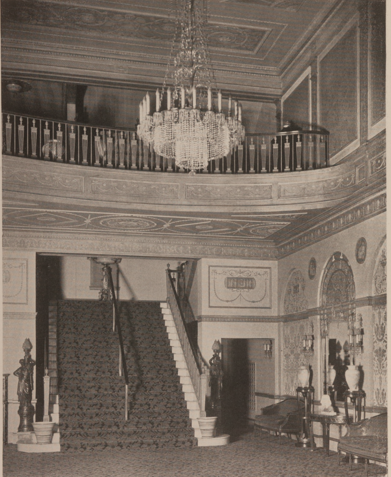
Staircase to Mezzanine Floor in the Capitol Theatre, Atlanta, Georgia
