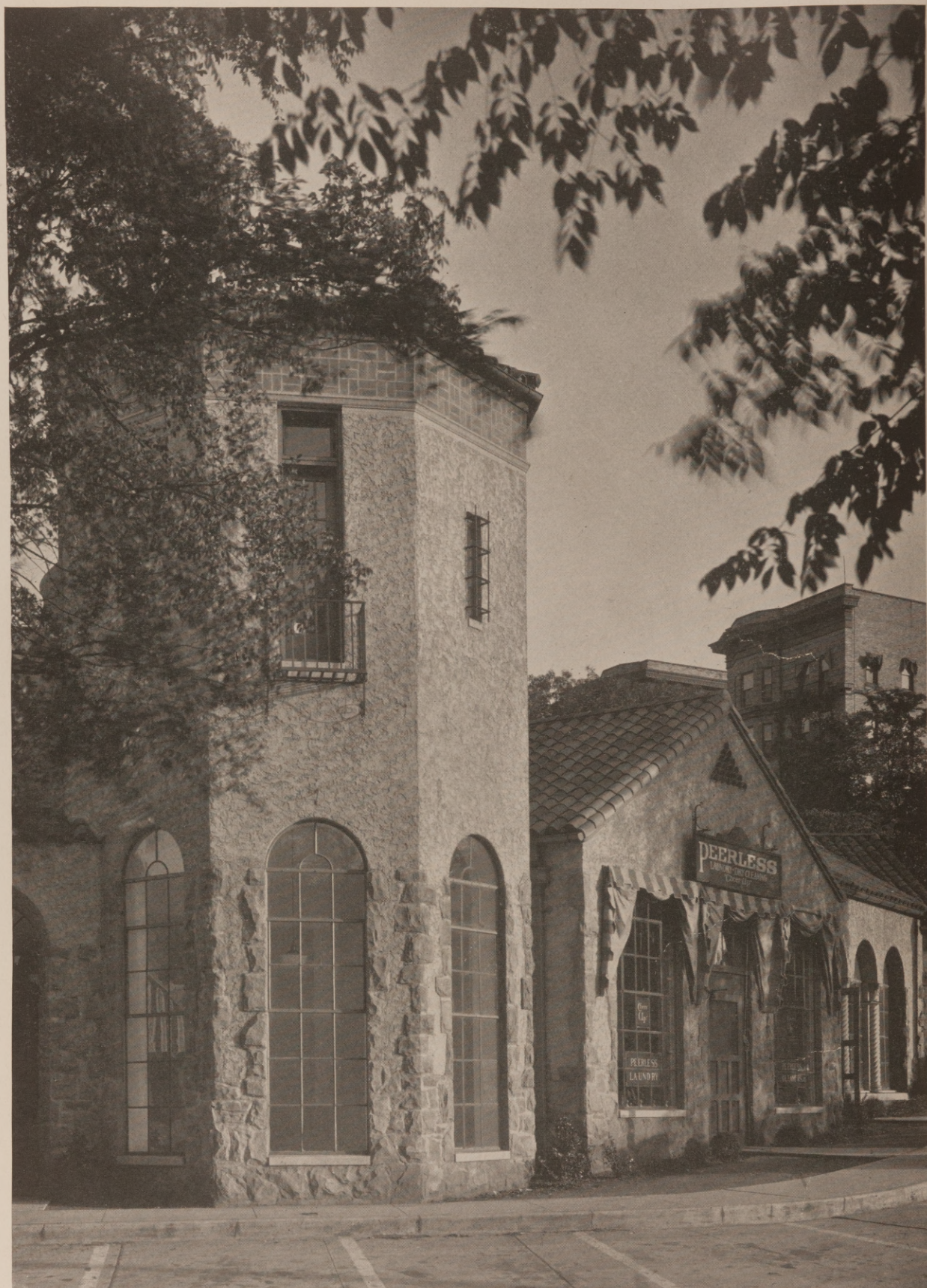
TOWER DETAIL, FIVE POINTS STORE GROUP, BIRMINGHAM, ALABAMA
