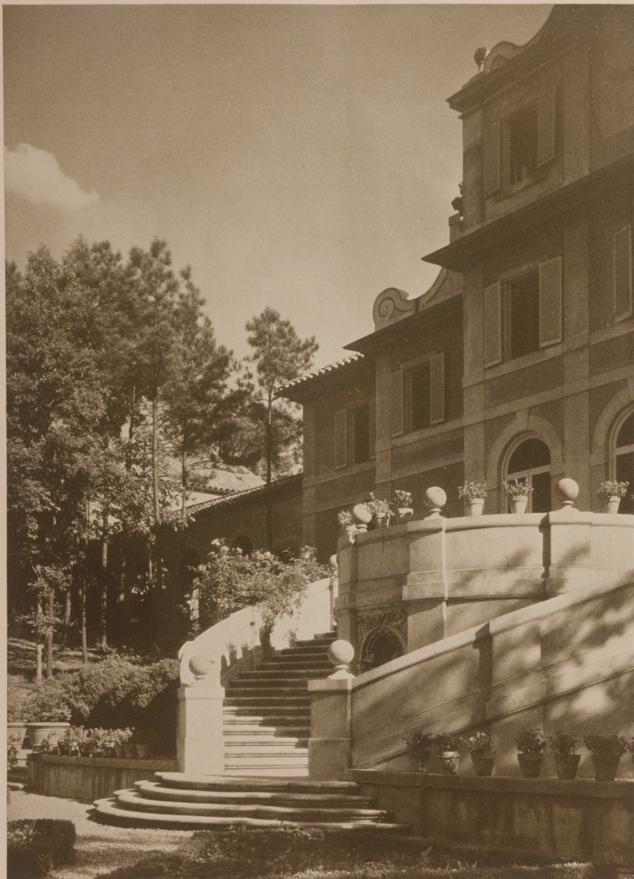
DETAIL OF GARDEN STAIR HOUSE OF ANDREW CALHOUN, ESQ., ATLANTA, GA. HENTZ, ADLER & SHUTZE, ARCHITECTS
