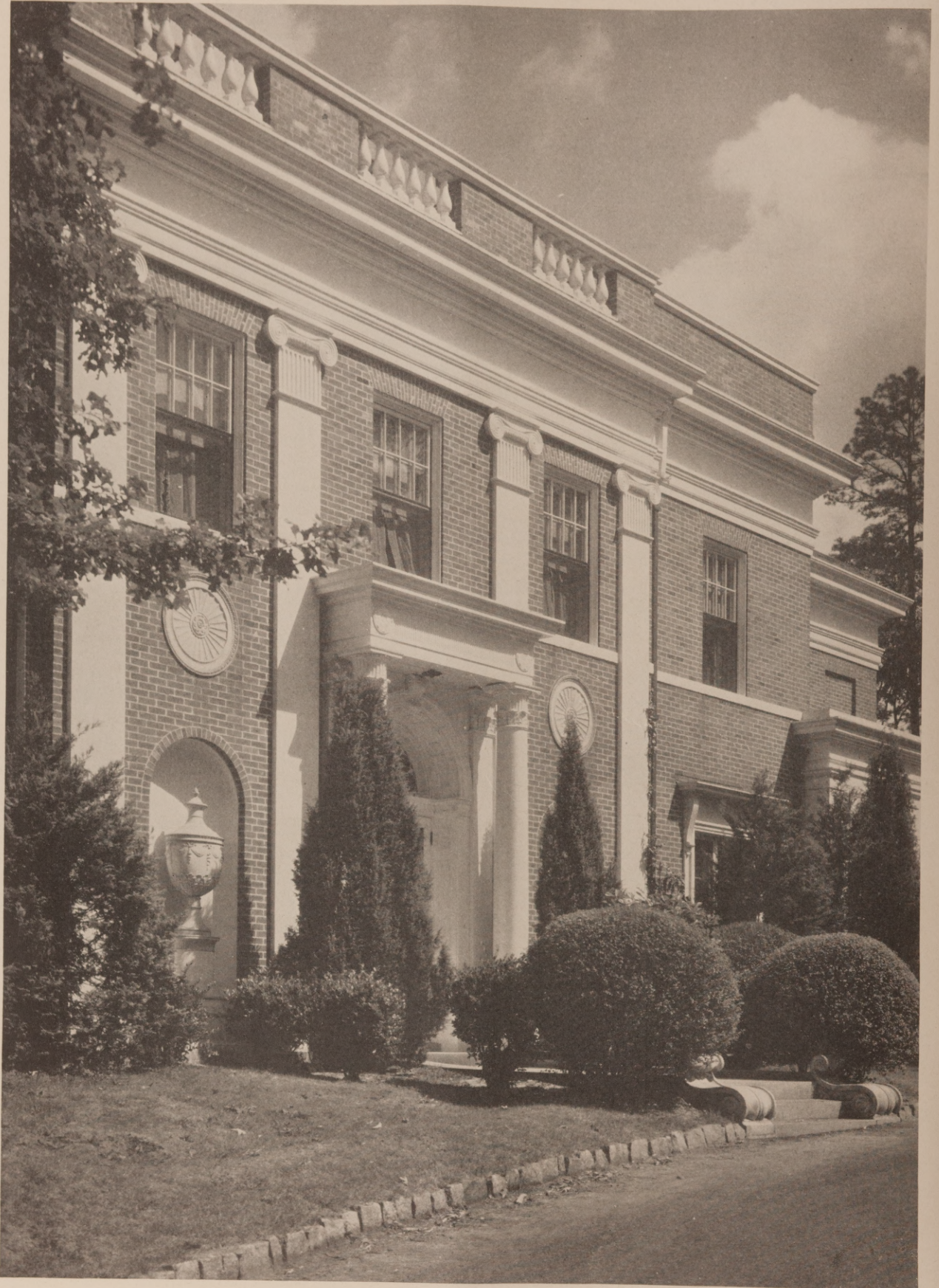
ENTRANCE DETAIL HOUSE OF PHILIP C. McDUFFIE, ESQ., ATLANTA, GA. HENTZ, ADLER & SHUTZE, ARCHITECTS
