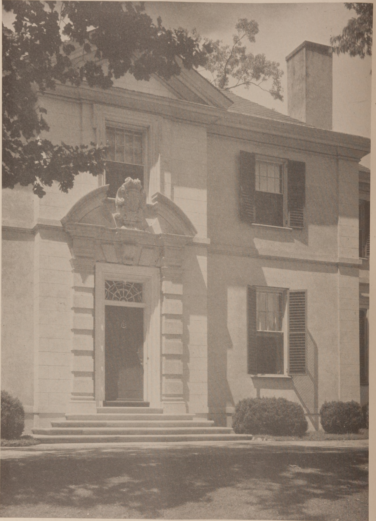
ENTRANCE DETAIL HOUSE OF HENRY TOMPKINS, ESQ., ATLANTA, GA. HENTZ, ADLER & SHUTZE, ARCHITECTS
