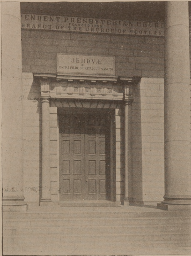
Entrance to Independent Presbyterian Church, Savannah.
