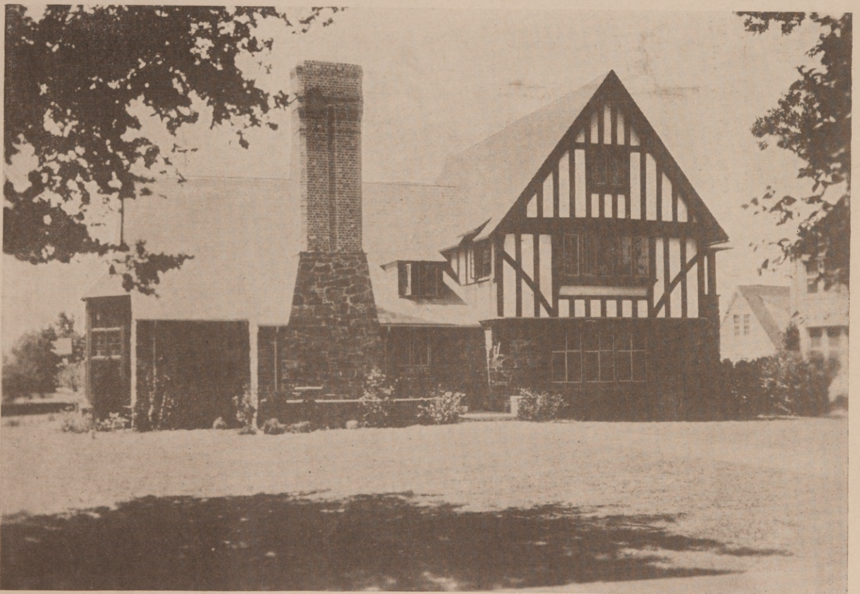
HOUSE OF MR. ANTON F. KORN, JR., DALLAS, TEXAS ANTON F. KORN, ARCHITECT.
