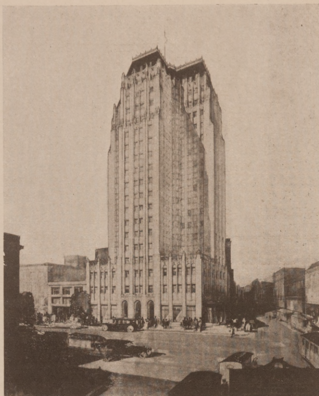
MEDICAL ARTS BUILDING, DALLAS, TEXAS C. E. BARGLEBAUGH, L. R. WHITSON AND F. O. DALE, ARCHITECTS.
