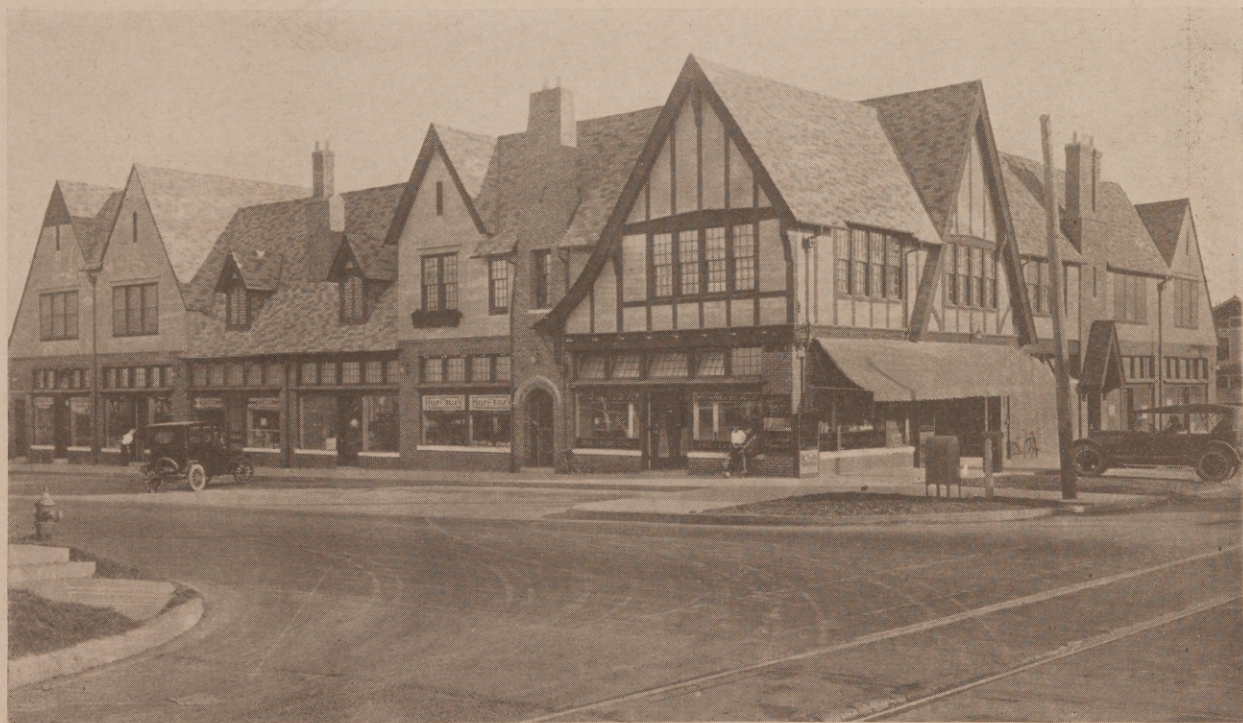
SUBURBAN SHOP AND OFFICE BUILDING, DALLAS, TEXAS FLINT & BROAD, ARCHITECTS
