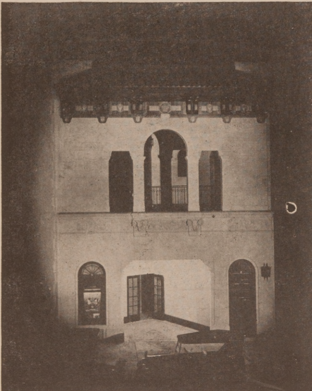
NORTH VIEW, DALLAS ATHLETIC CLUB BUILDING, DALLAS, TEXAS DUDLEY S. GREEN AND RALPH BRYAN, ARCHITECTS
