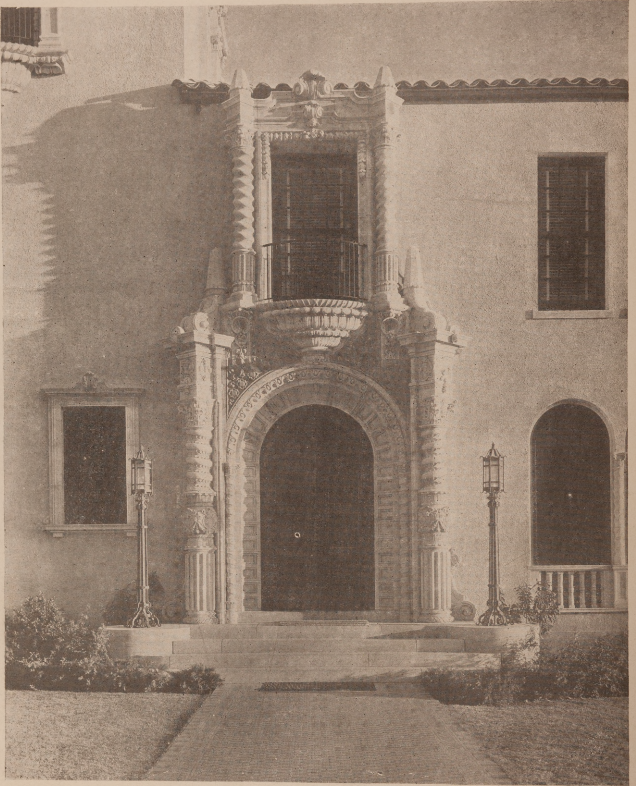
ENTRANCE DETAIL HIGHLAND PARK TOWN HALL, DALLAS, TEXAS LANG & WITCHELL, ARCHITECTS
