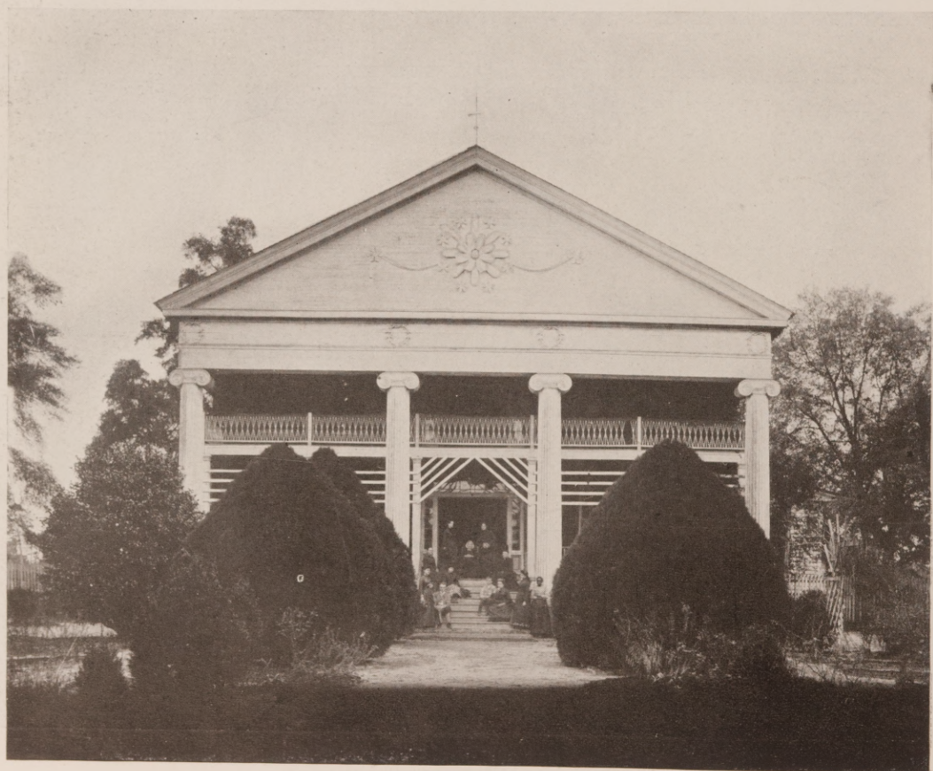
VIEW OF HOUSE THIRTY-FIVE YEARS AGO.
