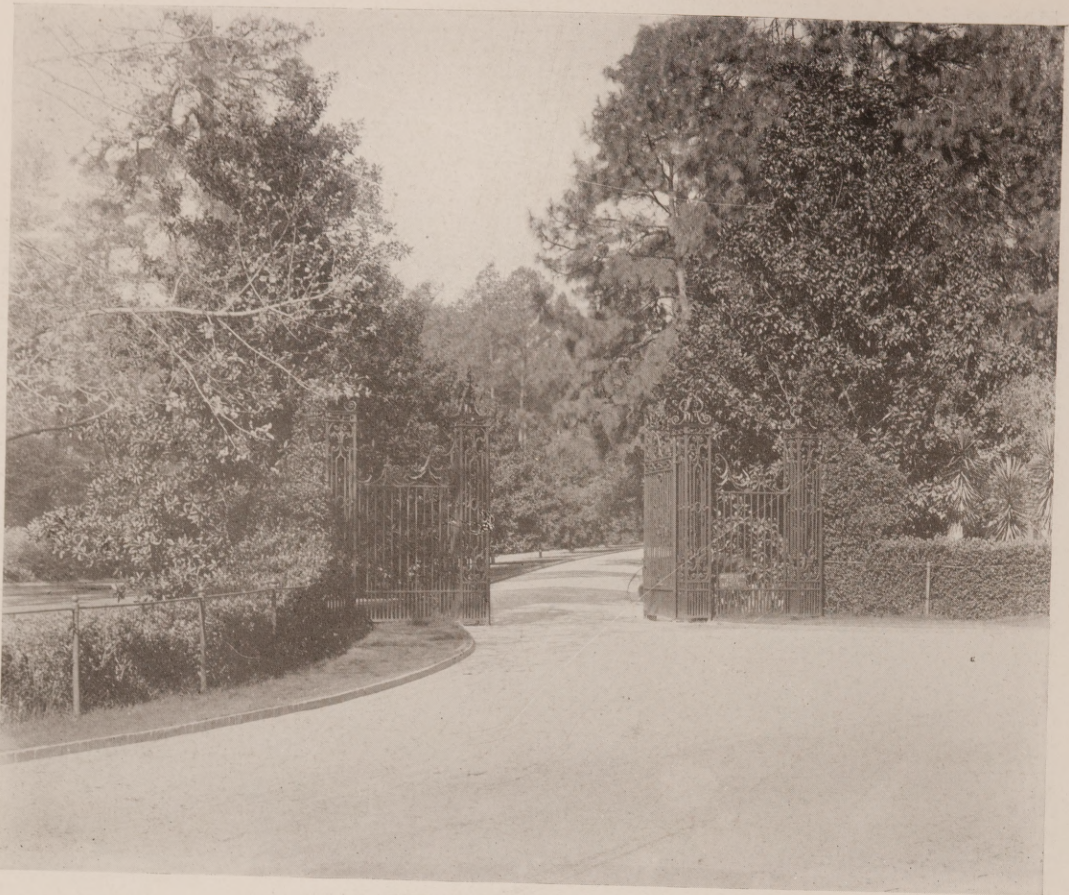
VIEW OF ENTRANCE GATEWAY.
