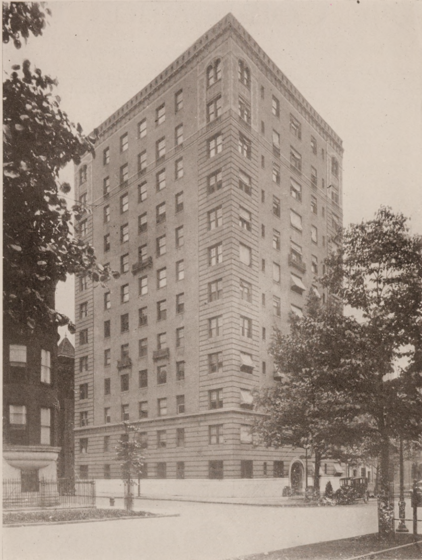
TWELVE-STORY ELEVATED APARTMENT 270 WEST END AVE., NEW YORK CITY
