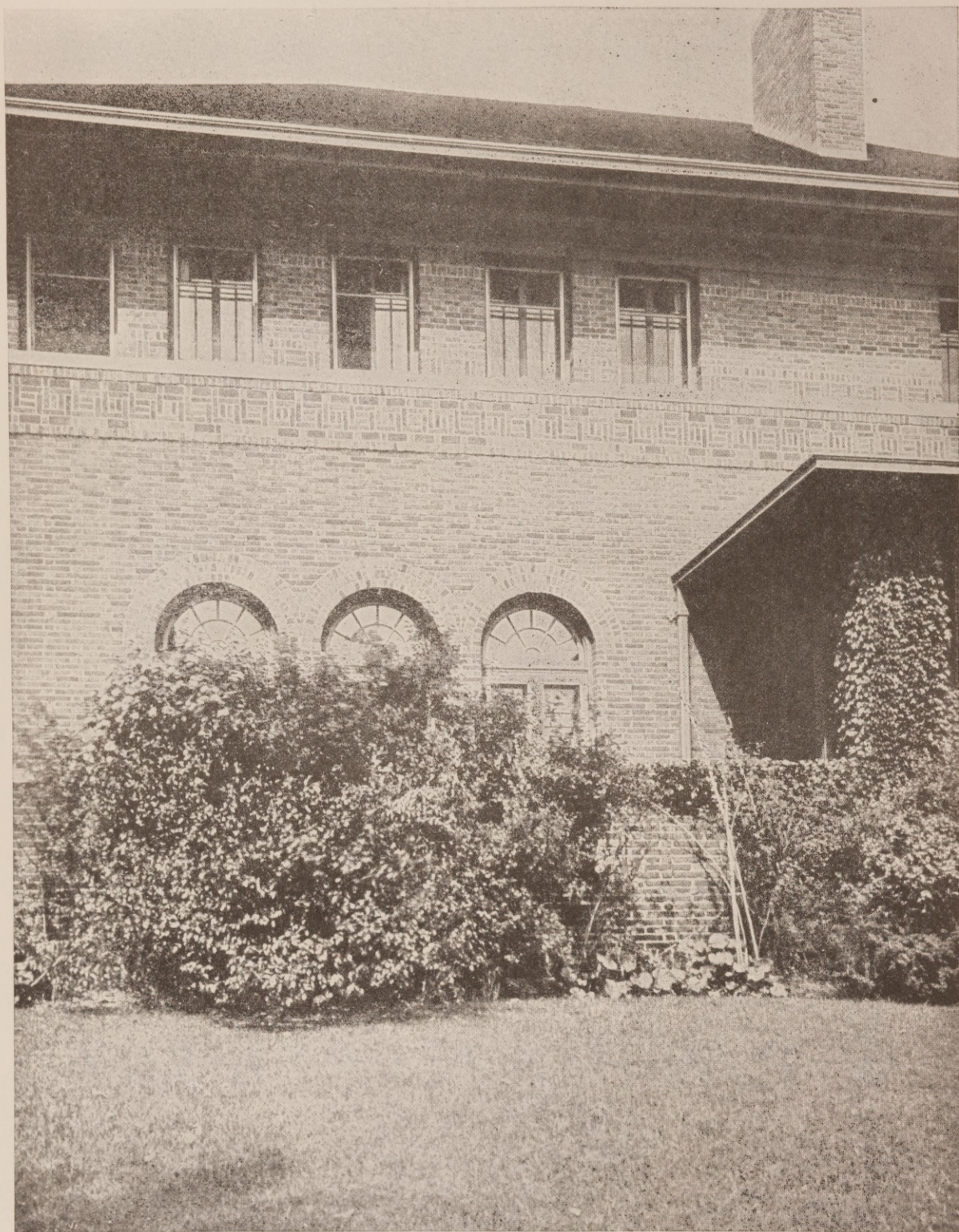
Detail of Residence, Evanston, Illinois. Perkins, Fellows & Hamilton, Architects
