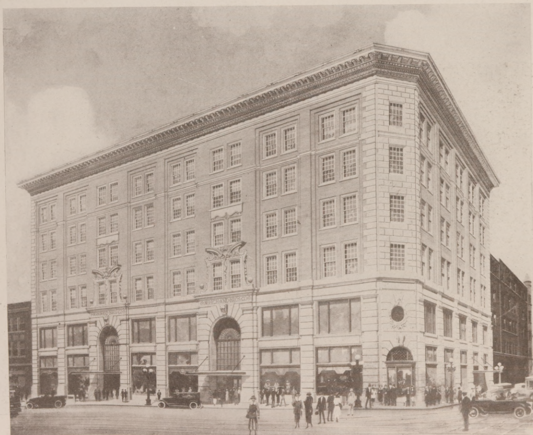
BUILDING FOR M. RICH & BROS. CO., ATLANTA, GA. HENTZ, REID & ADLER, ARCHITECTS.
