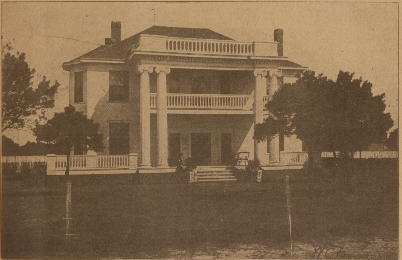
One of the Few Colonial Residences at Pensacola, Fla. W. C. Frederic, Architect.
