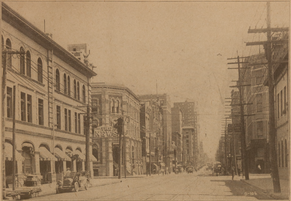
View of Commerce Street in Dallas Looking East.
