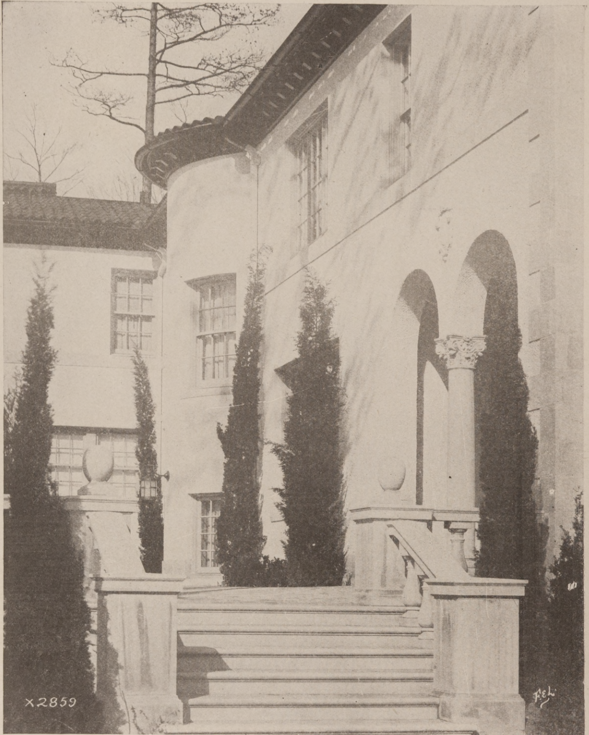
ENTRANCE GARDEN SIDE HOUSE OF HAROLD ROGERS, ESQ., ATLANTA, GA. PRINGLE & SMITH, ARCHITECTS.
