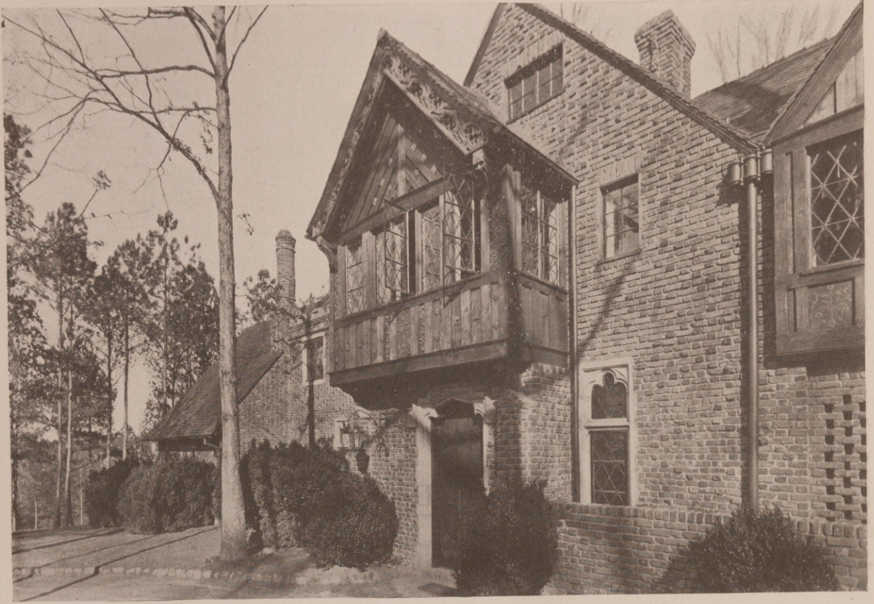
REAR ENTRANCE DETAIL
