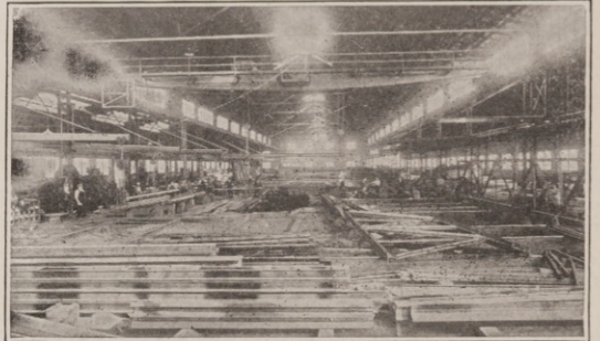
INTERIOR VIEW OF OUR STRUCTURAL STEEL PLANT.
