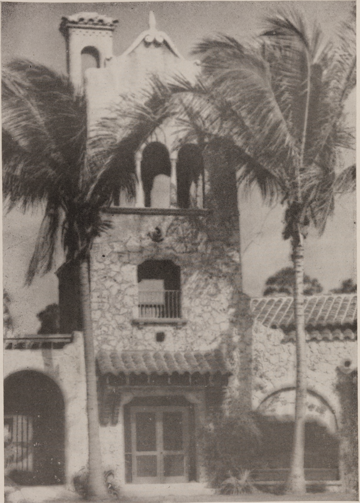
DETAIL OF TOWER CORAL GABLES COUNTRY CLUB, MIAMI, FLA. M. L. HAMPTON, ARCHITECT.
