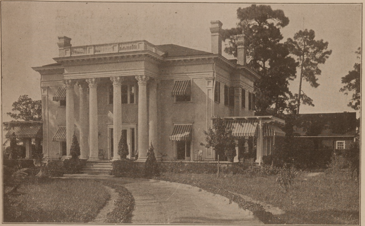
Hofe of Wm. H. Fleming, Augusta, Ga. W. T. Downing, Architect, Atlanta, Ga.
