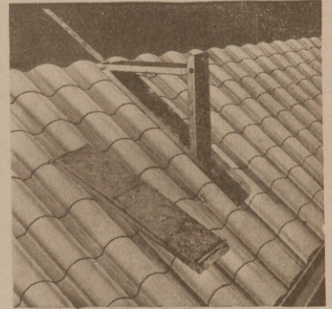
Spanish Tile Roof.
