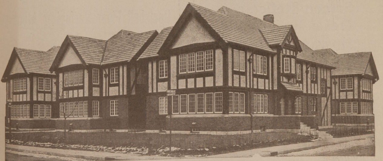
Eight apartment building, corner Maple Boulevard and Delaware St., Indianapolis, Ind. Roofed by Gibraltar Concrete Co., with "Walter Concrete tile." Perry E. Powell, owner and builder.
