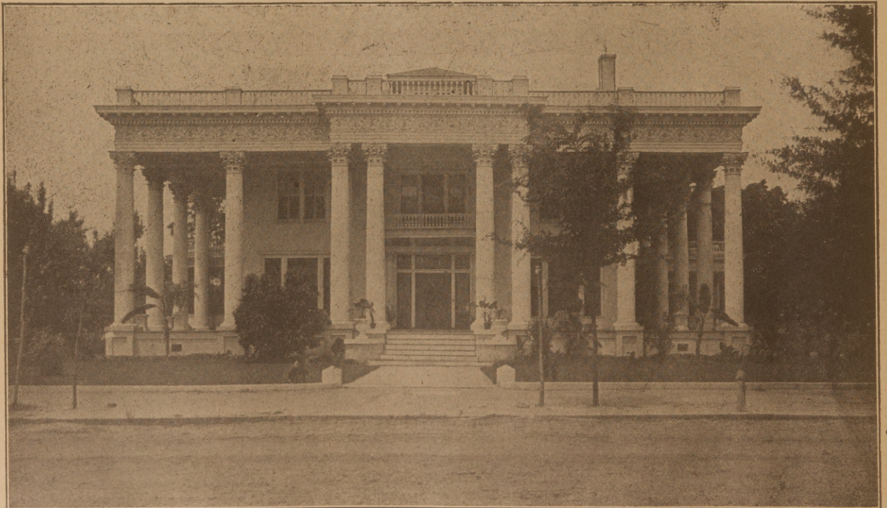
Residence of Hon. E. S. Shorter, Eufaula, Ala. C. R. Ellis, Architect.
