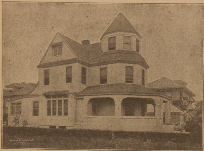
Radiant shingles over old wood shingles.
