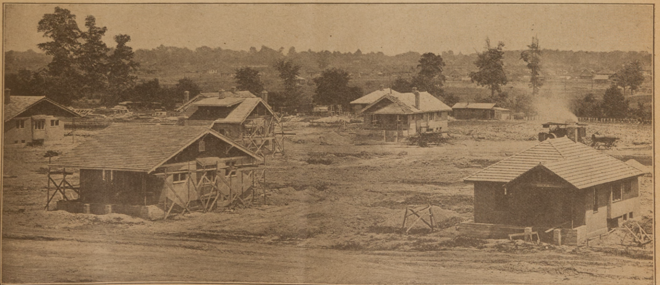
Houses for Lafayette Motors Employees. Roofed with Concretile. J. Edwin Kopf, Architects.
