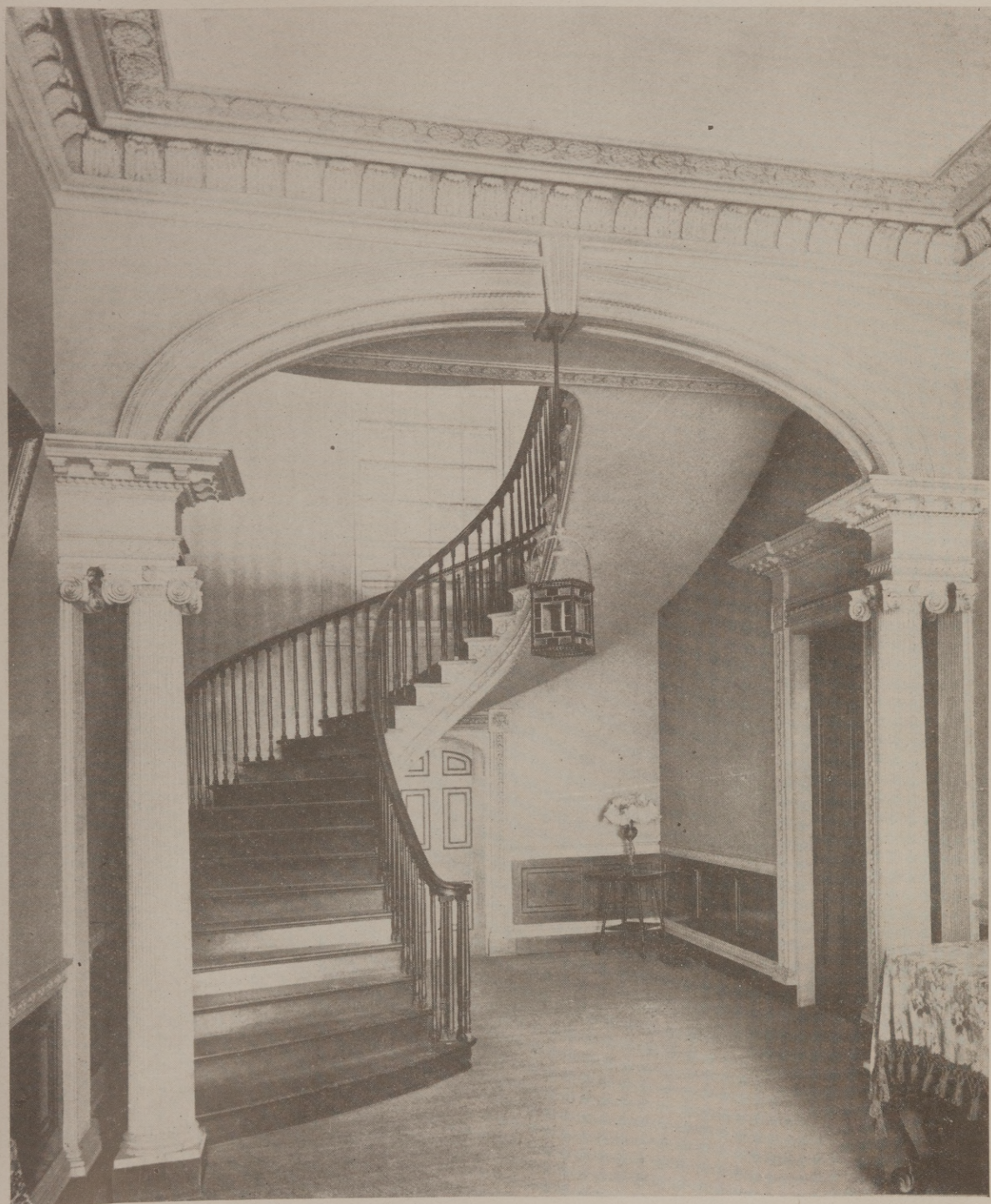
DETAIL STAIRWAY BENNET HOUSE, CHARLESTON, S. C. BUILT 1767.
