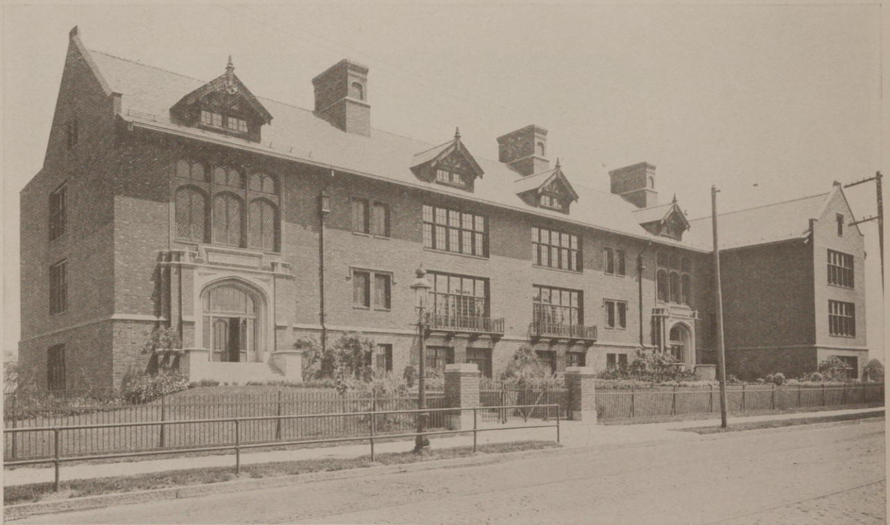
The Isaac M. Mason School for elementary pupils. The building is so erected that another wing may be added. This is a provision in many of the St. Louis schools so that increased attendance may be accommodated without planning a new building.
