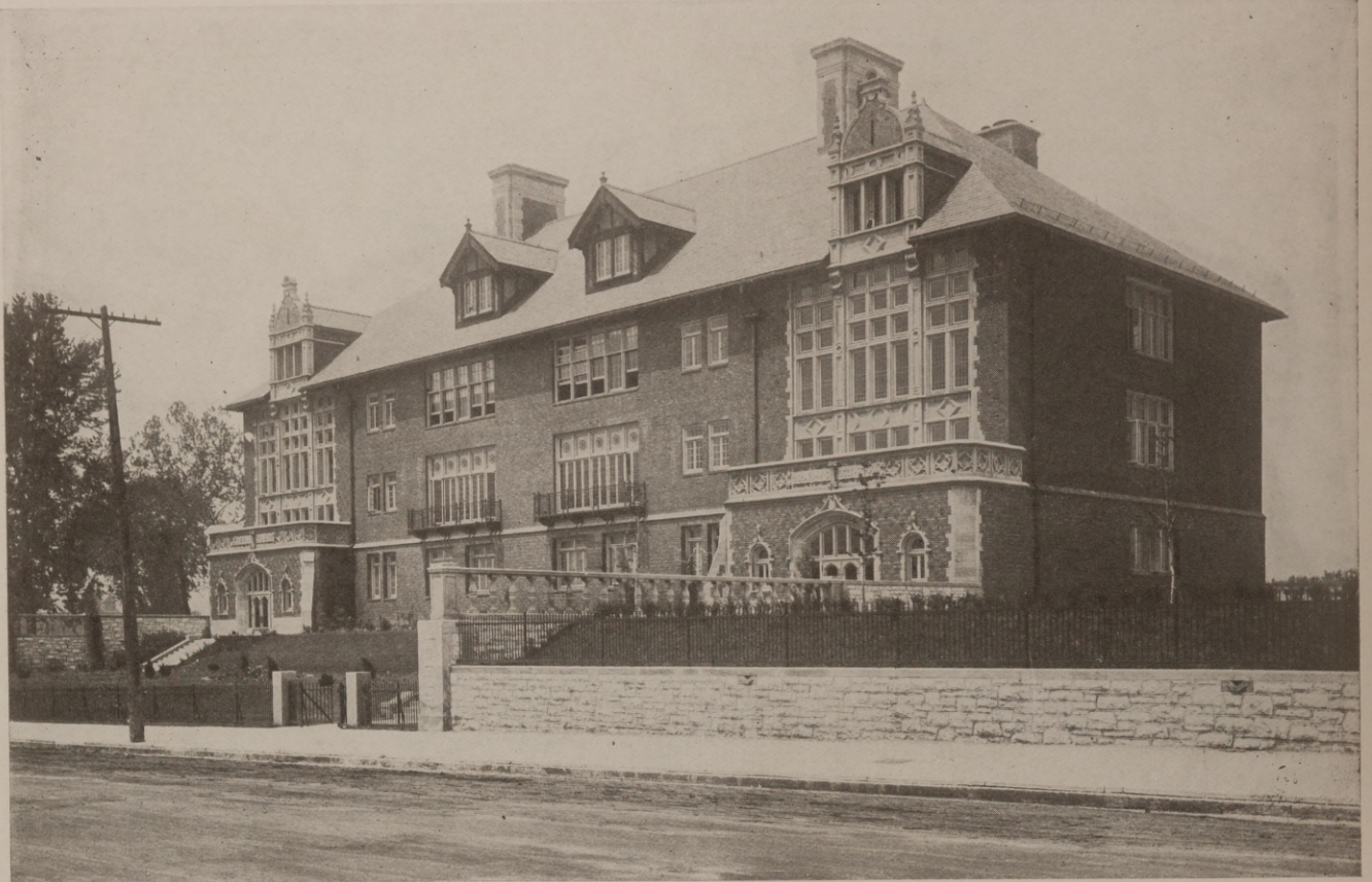
The Richard M. Scruggs School, which has two ornamental entrances with a perfect balance in architecture and design. The windows are set off to advantage by the trim of white stone that affords a contrast to the darker brick. All St. Louis school buildings are of brick, concrete and steel, affording a fireproof structure.
